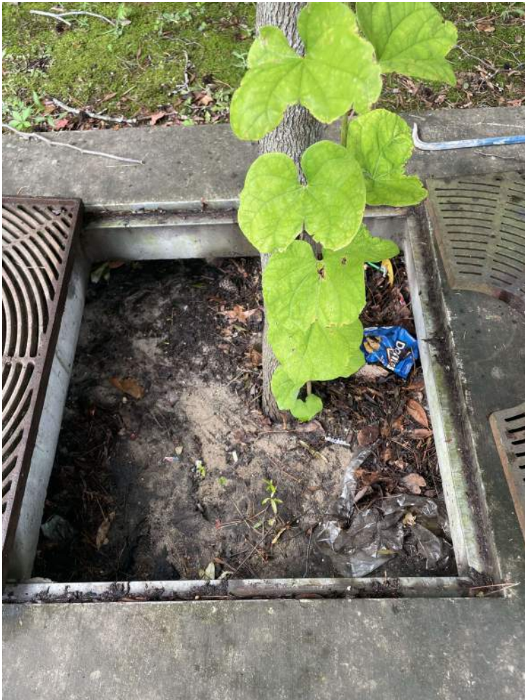
BMP #11- before maintenance
