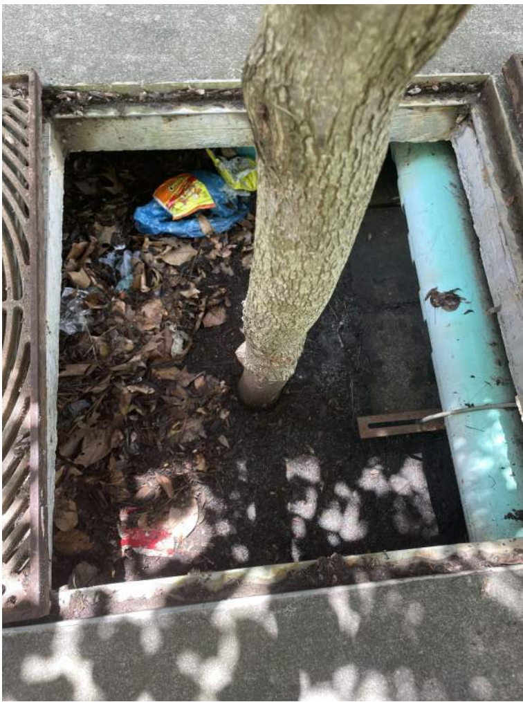
BMP #16- before maintenance
