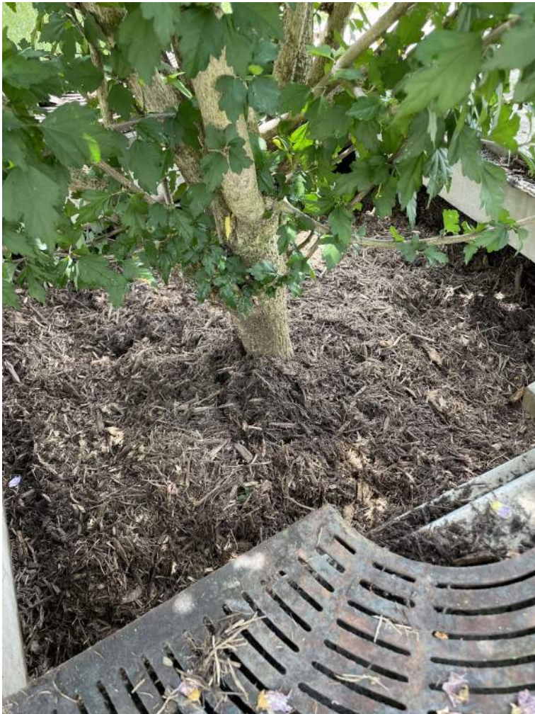
BMP #42- after maintenance
