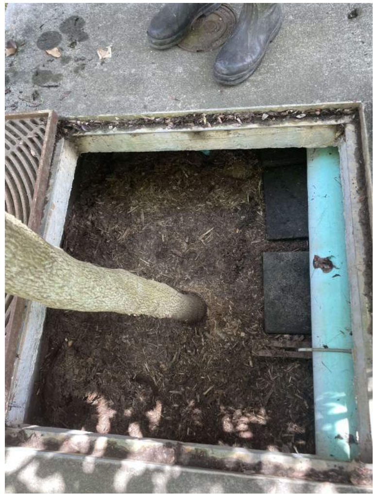
BMP #16- after maintenance
