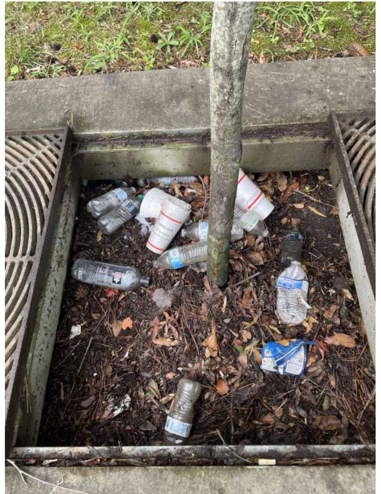
BMP #11- before maintenance
