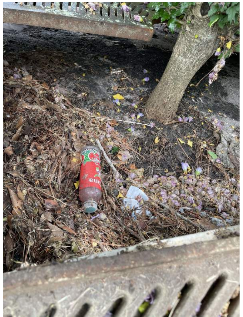
BMP #42- before maintenance
