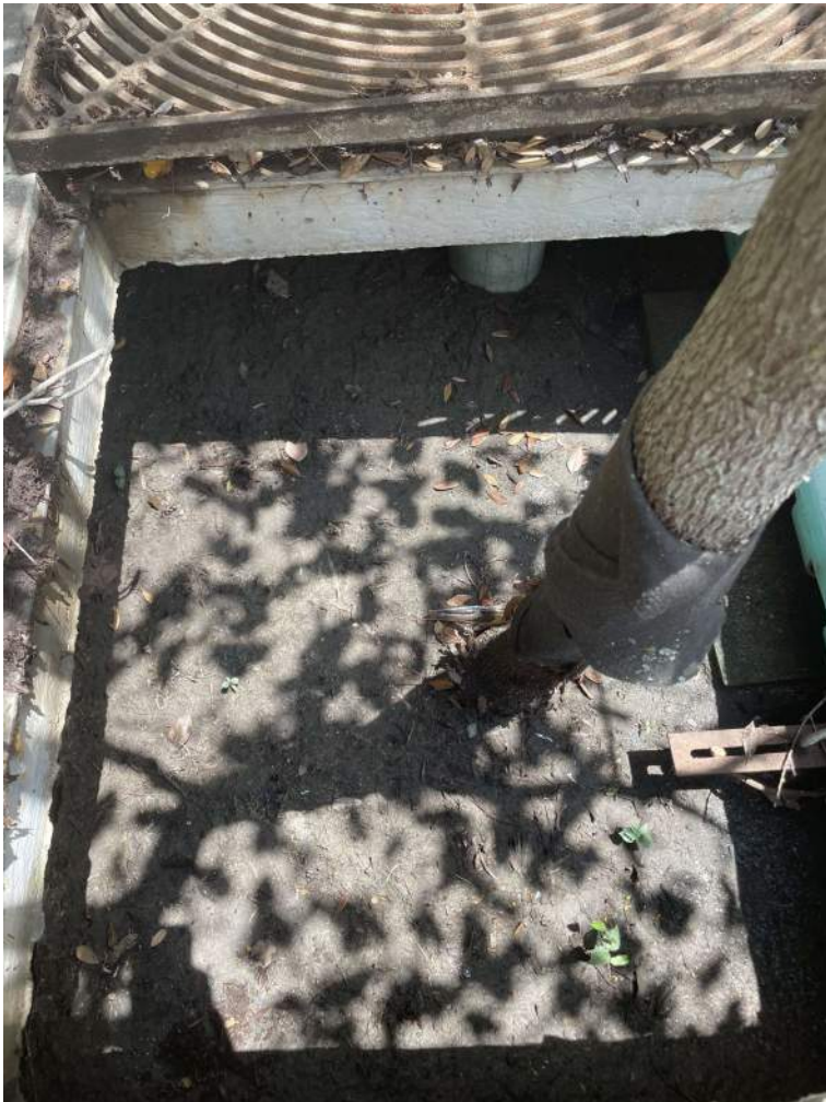
BMP #21- before maintenance
