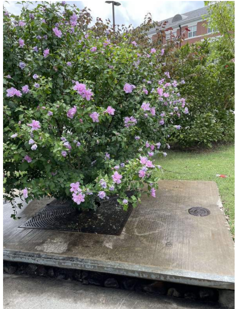
BMP #42- after maintenance
