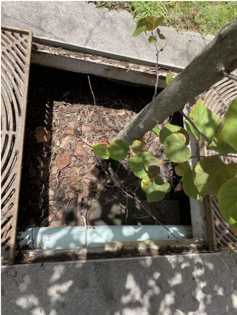
BMP #4- before maintenance
