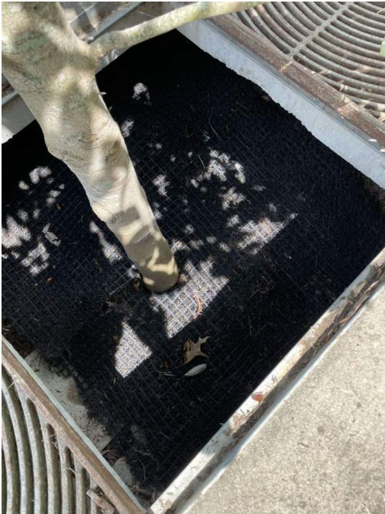
BMP #5- after maintenance
