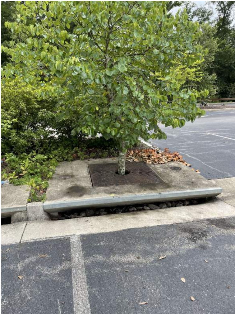
BMP #9- after maintenance
