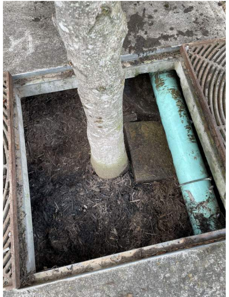
BMP #18- after maintenance
