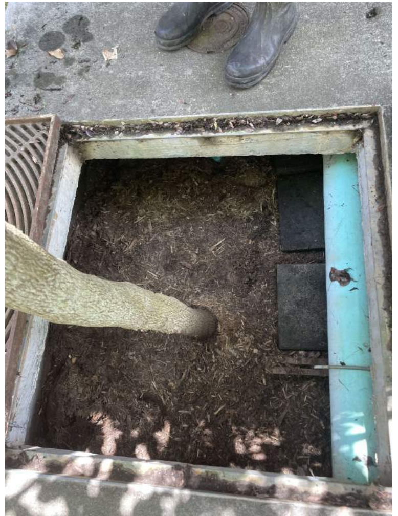
BMP #21- after maintenance
