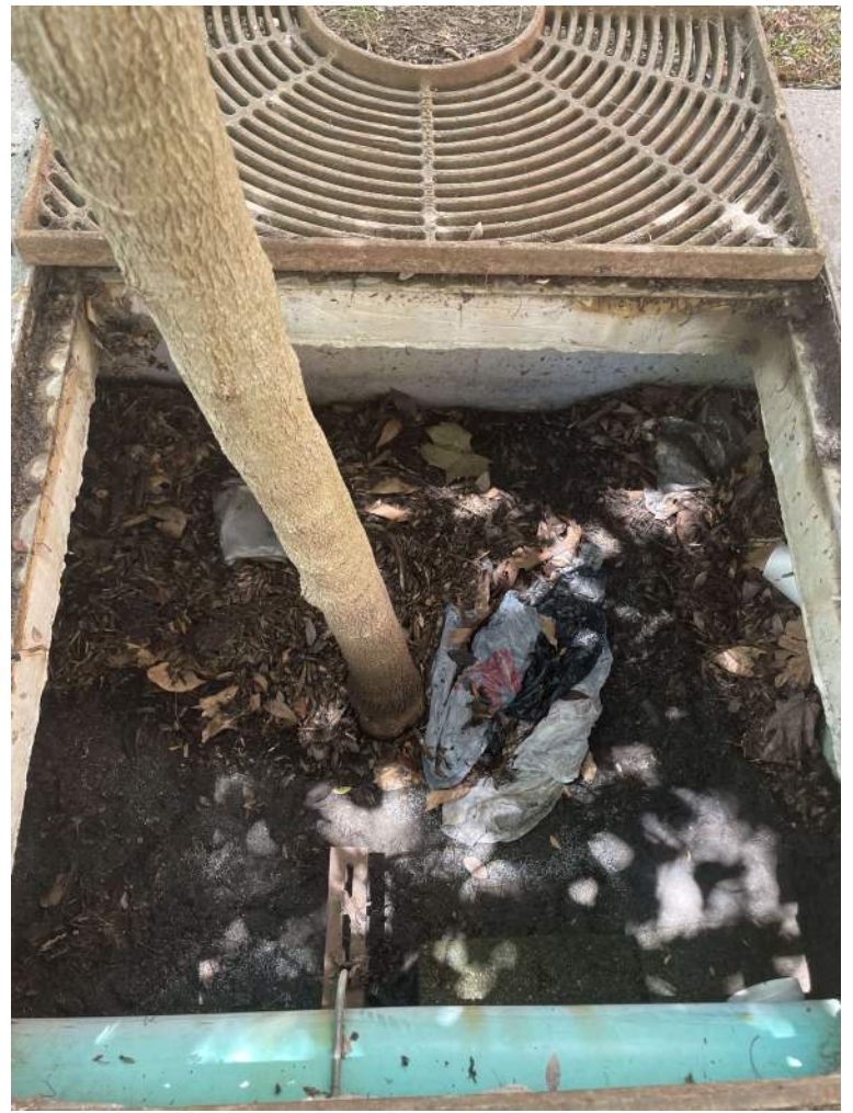
BMP#1- before maintenance
