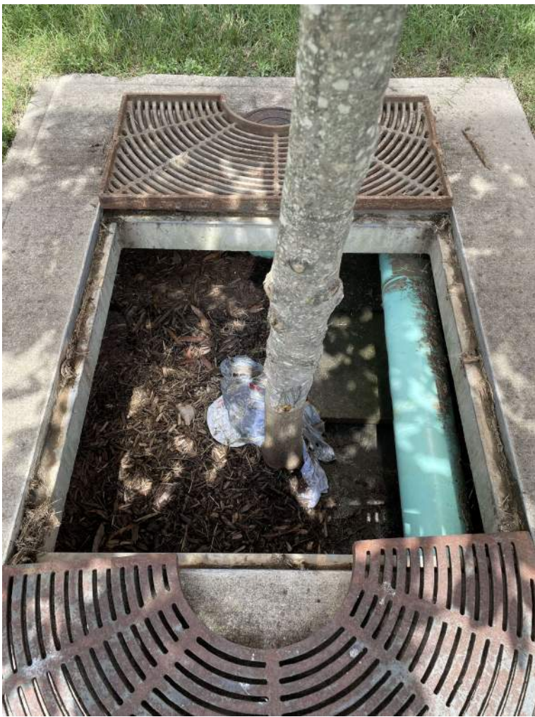
BMP #6- before maintenance
