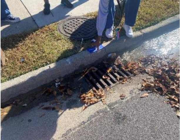
Figure 2. Storm Drain Marking
