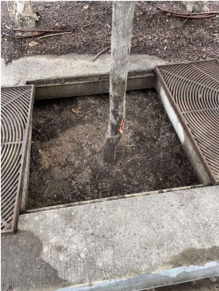
BMP #8- after maintenance
