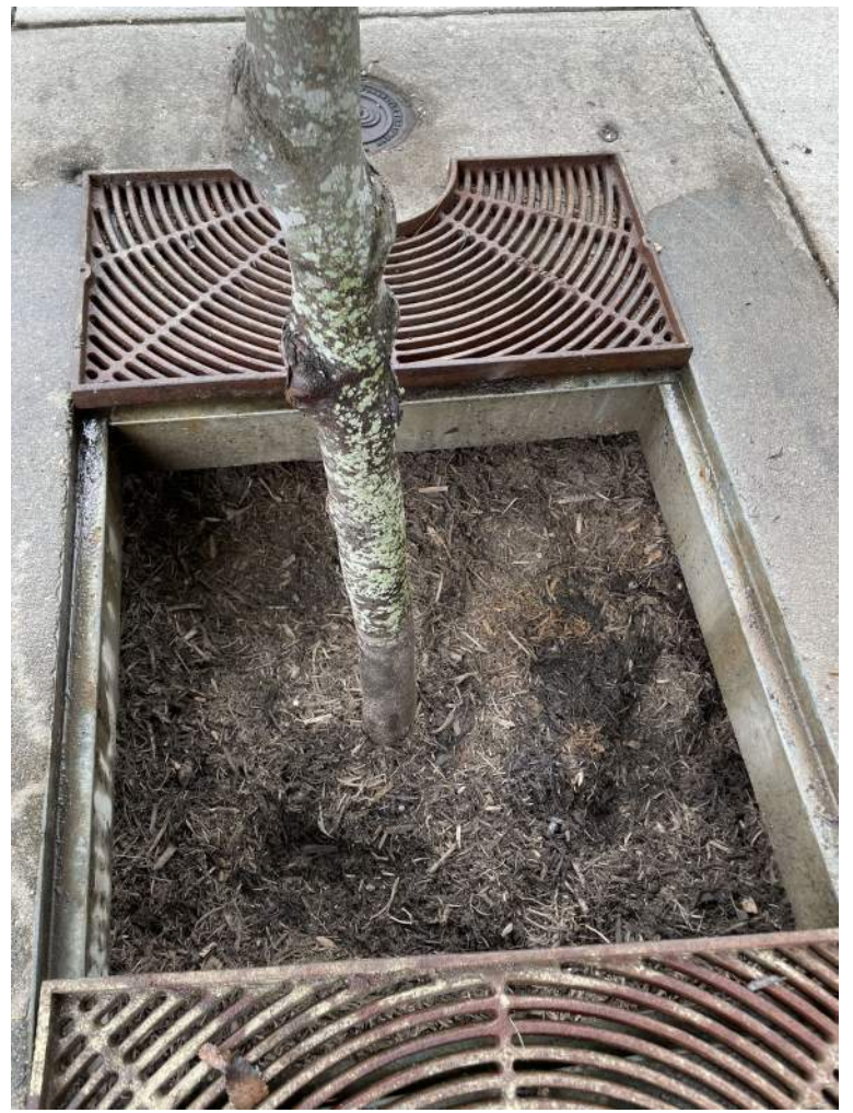
BMP #12- after maintenance
