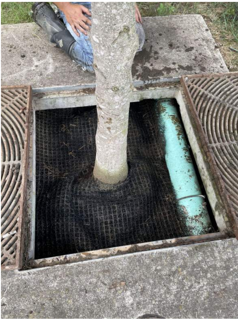
BMP #18- after maintenance
