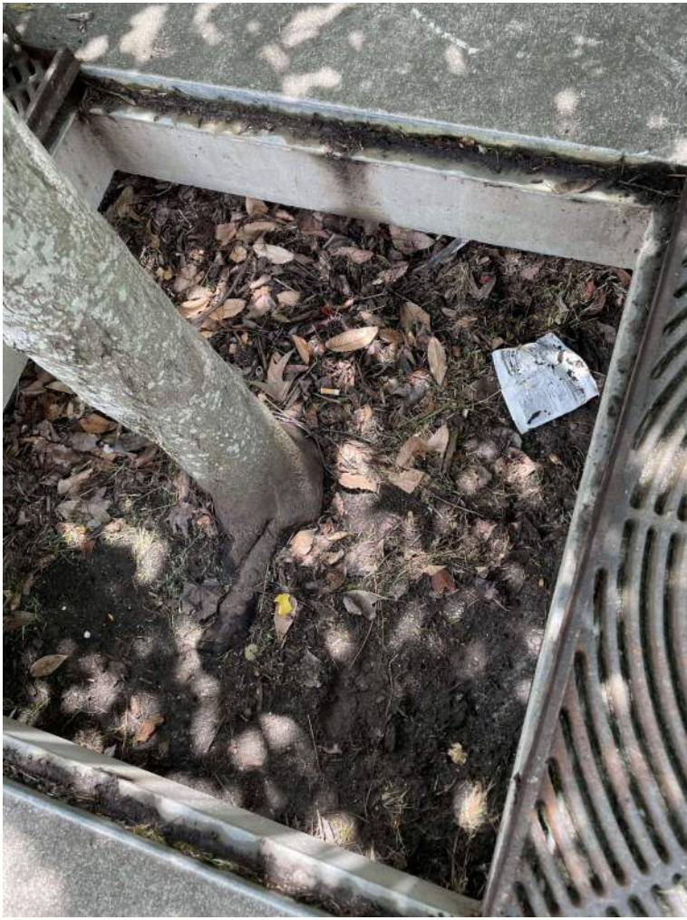
BMP #13- before maintenance
