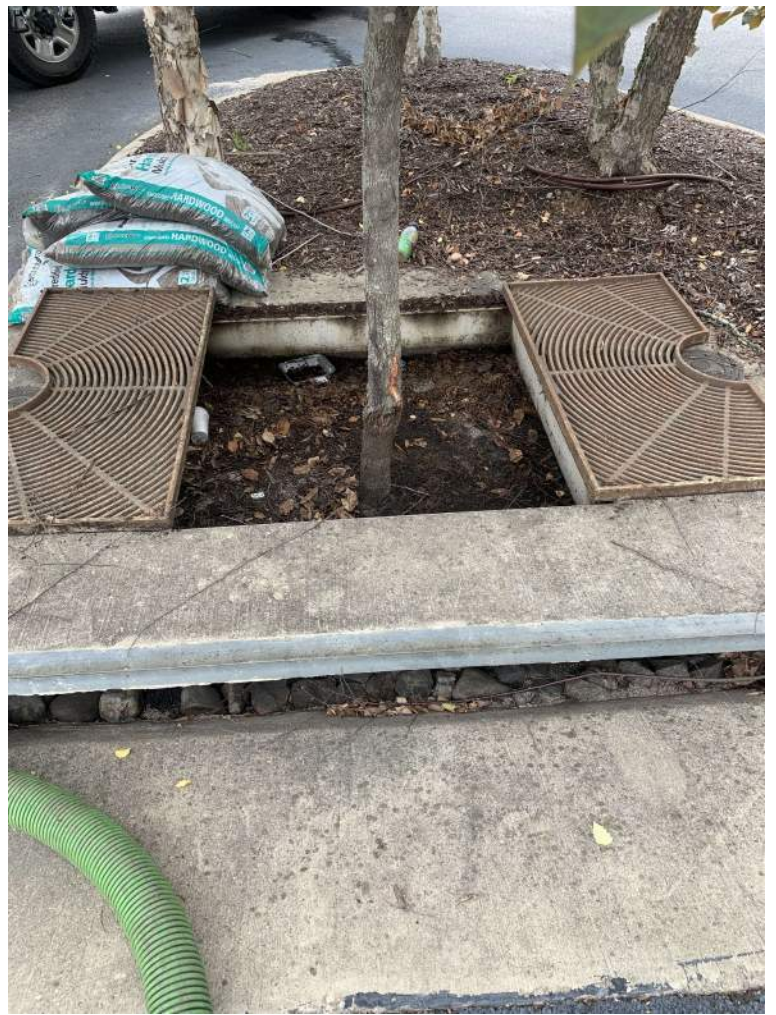
BMP #8- before maintenance
