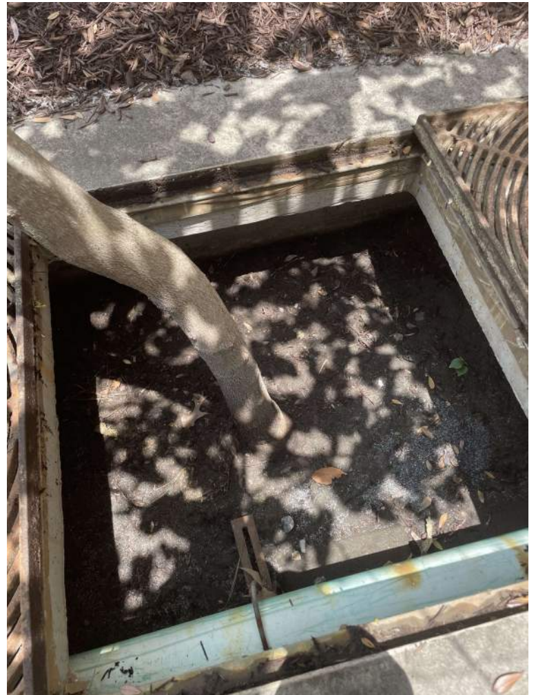
BMP #17- before maintenance
