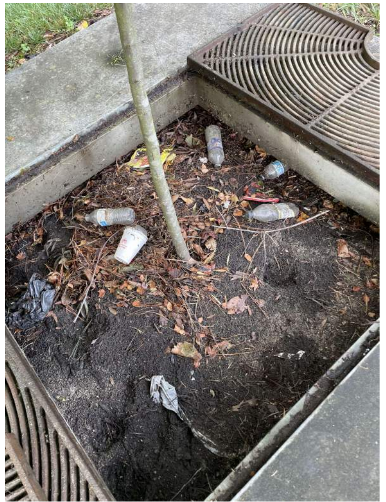
BMP #10- before maintenance
