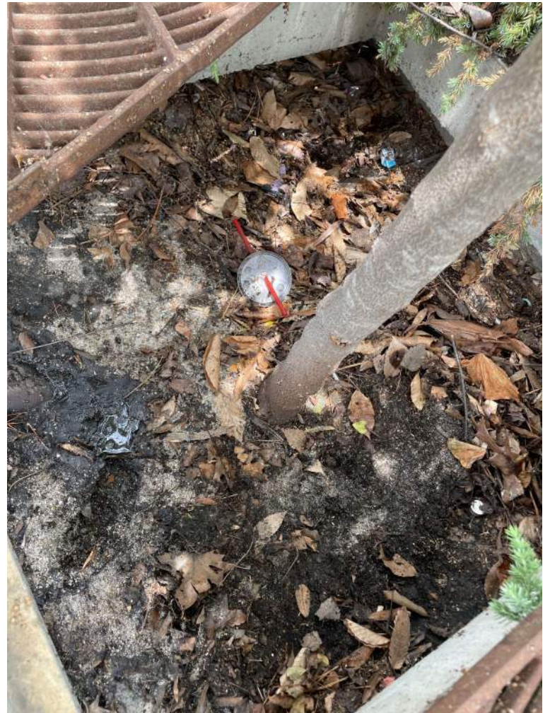
BMP #7- before maintenance
