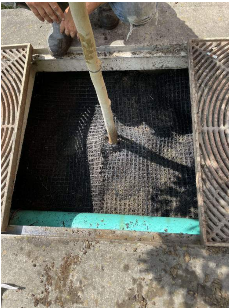
BMP #19- after maintenance
