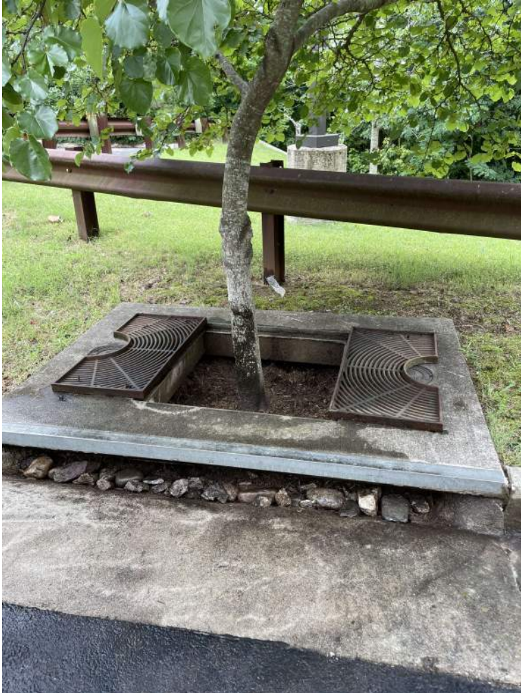
BMP #13- after maintenance
