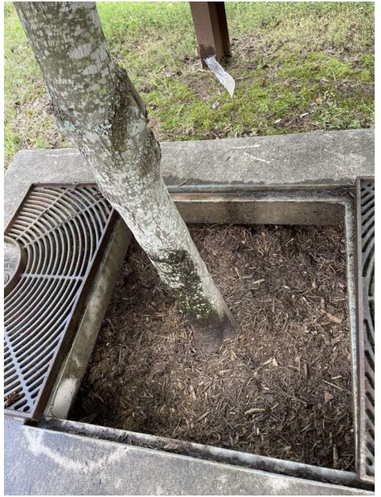
BMP #13- after maintenance
