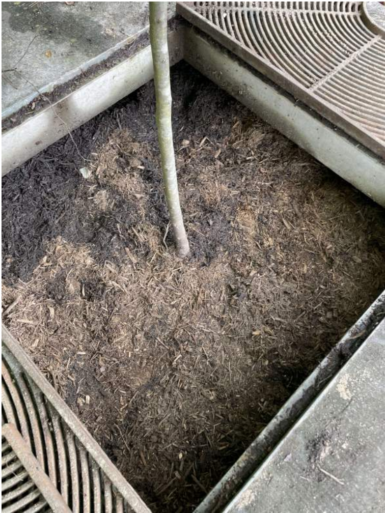
BMP #10- after maintenance
