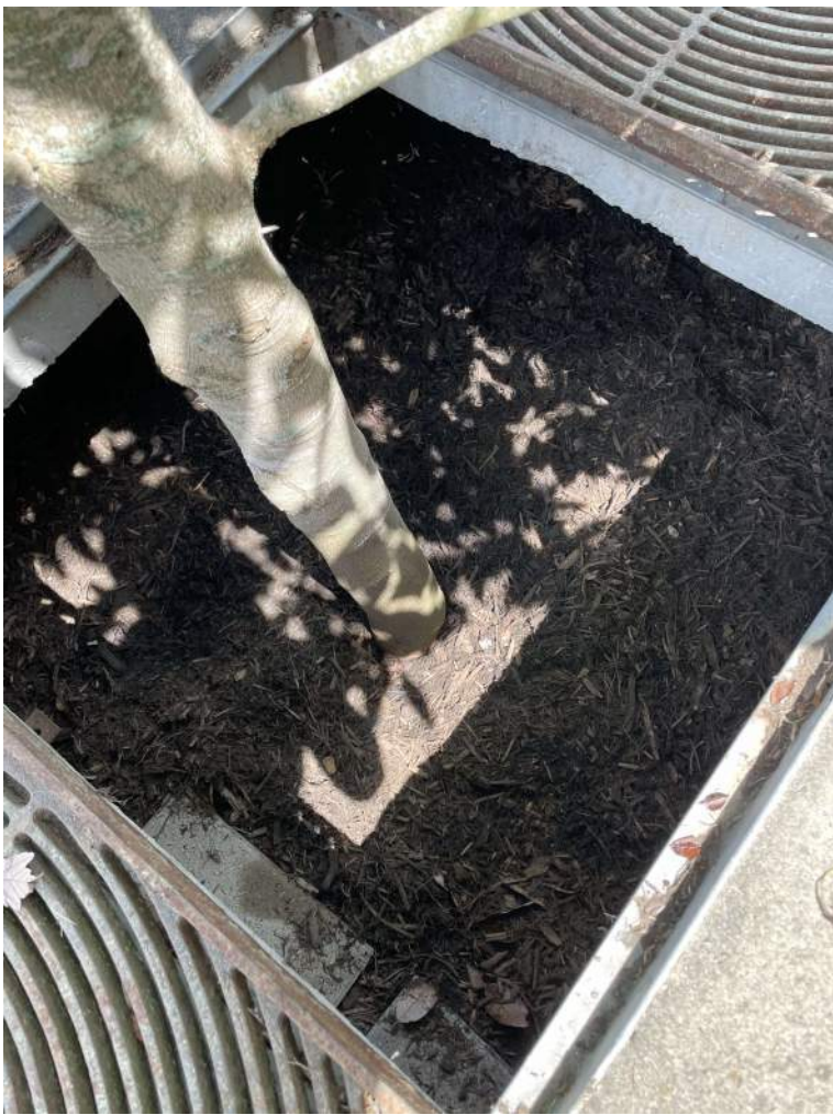
BMP #3- after maintenance
