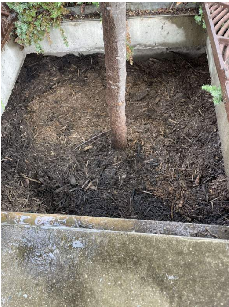
BMP #7- after maintenance
