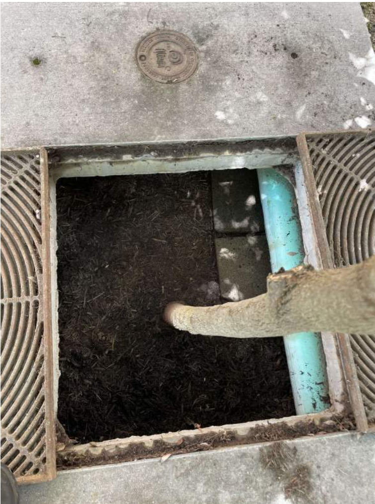
BMP #1- after maintenance
