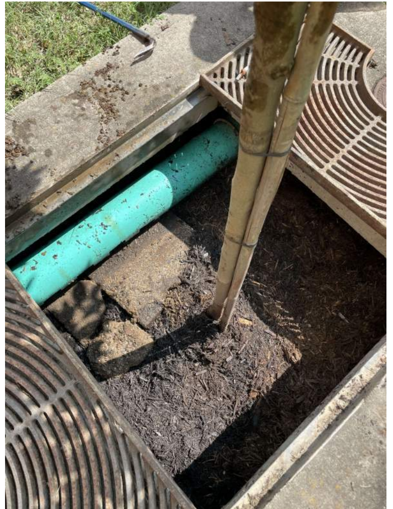
BMP #19- after maintenance
