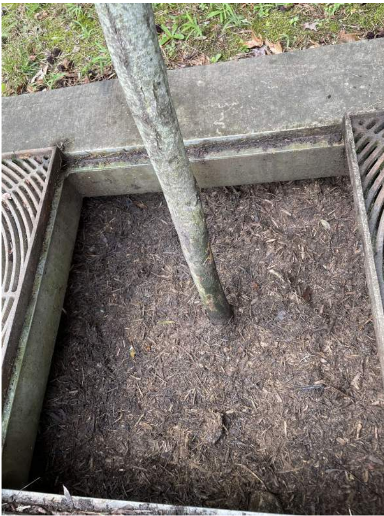
BMP #11- after maintenance
