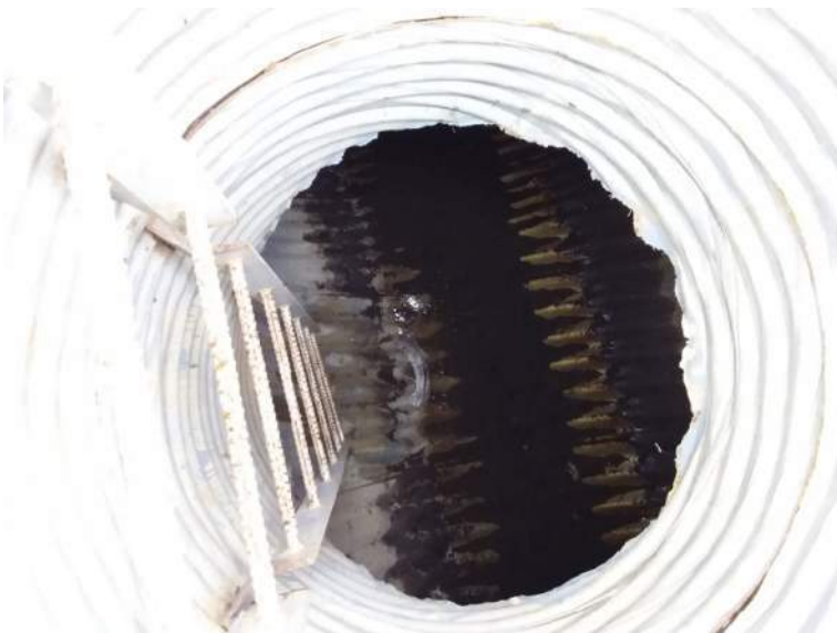
BMP #50- inside view
