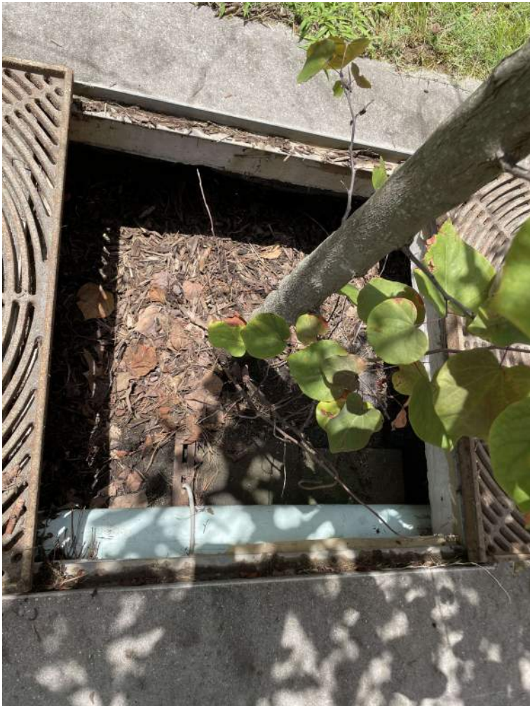
BMP #4- before maintenance
