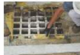
To remove Siltack®, clean area around grate and slide rebar through Siltack® pockets.
