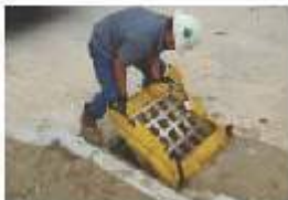
Replace Siltack® and grate inlet into recess.
