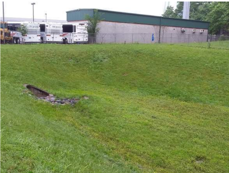
BMP #29- inlet area
