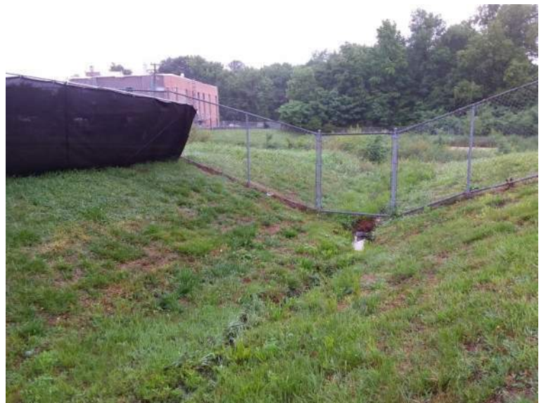
BMP #30- inlet channel
