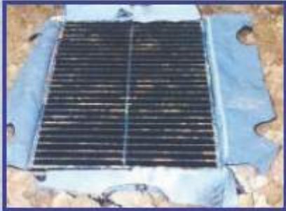
Installed Siltsack held in place by grate.
