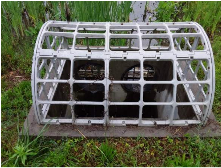
BMP #46- close up of outlet structure
