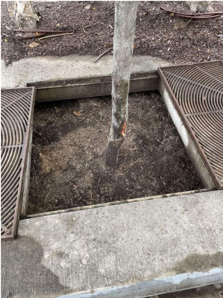
BMP #8- after maintenance
