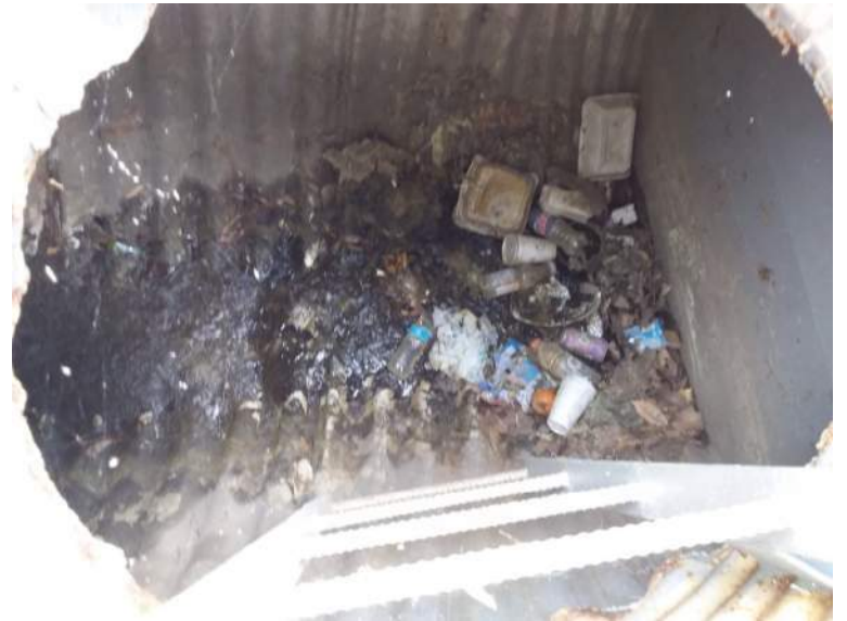
BMP #40- inside view of left manhole
