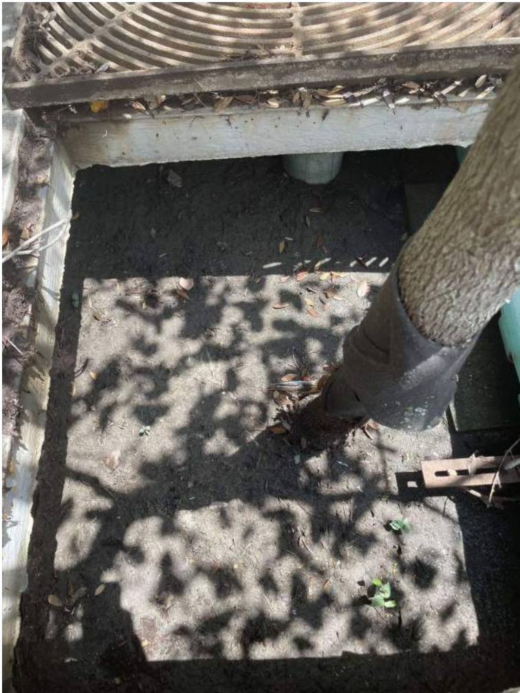
BMP #21- before maintenance
