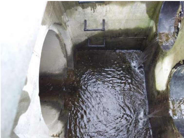
BMP #46- inside view of outlet structure
