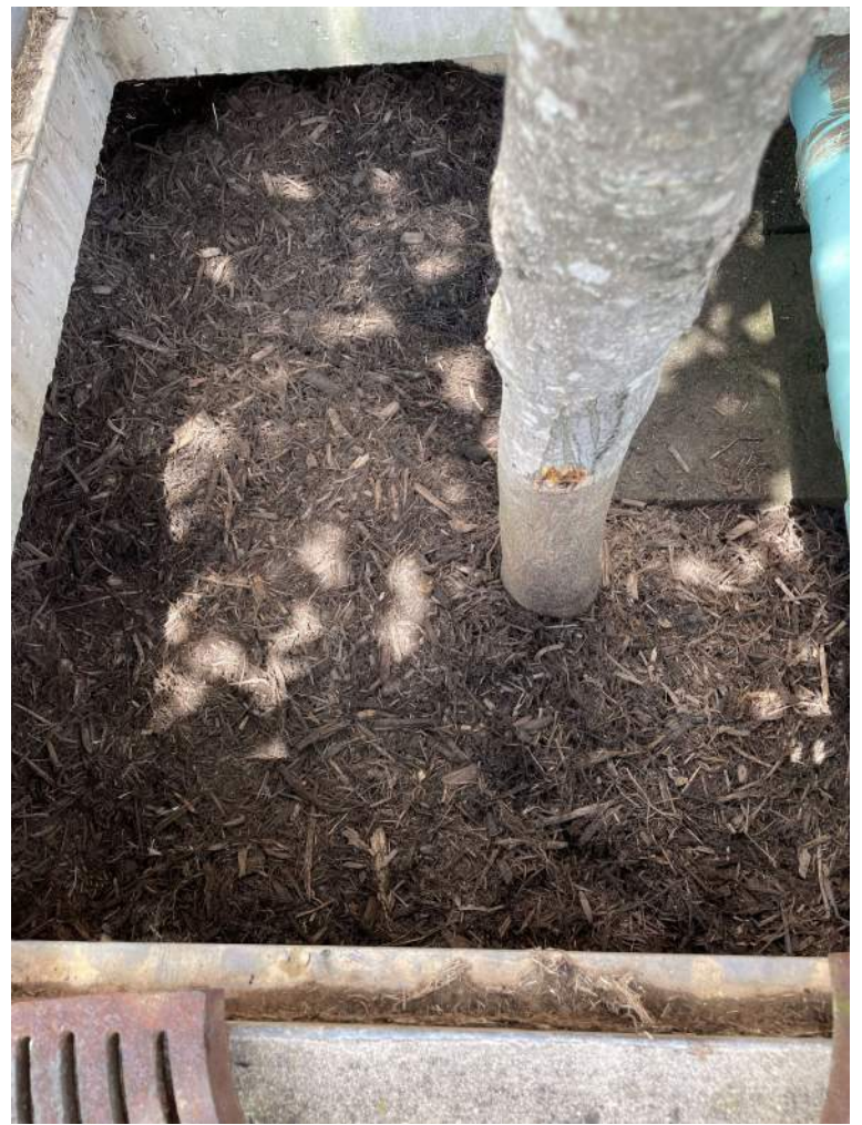
BMP #6- after maintenance
