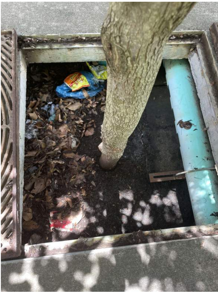
BMP #16- before maintenance
