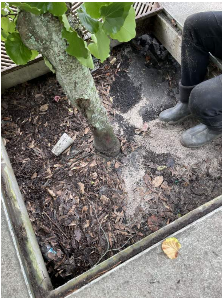
BMP #9- before maintenance
