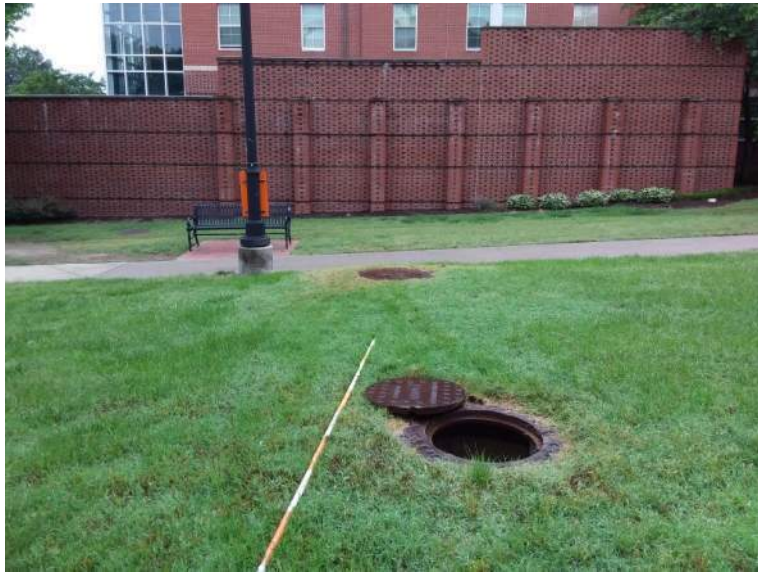
BMP #27- top view of sand filter side
