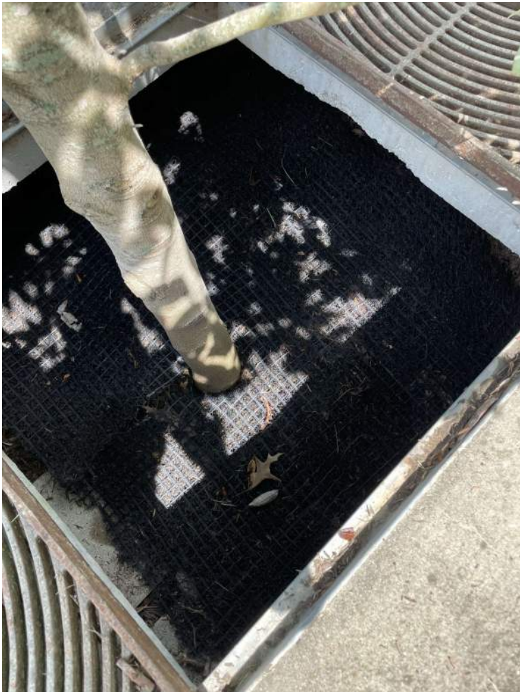
BMP #5- after maintenance
