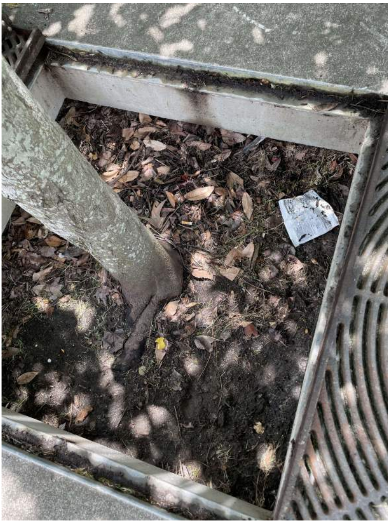
BMP #13- before maintenance
