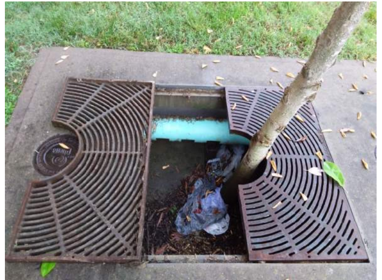
BMP #17- inside filterra
