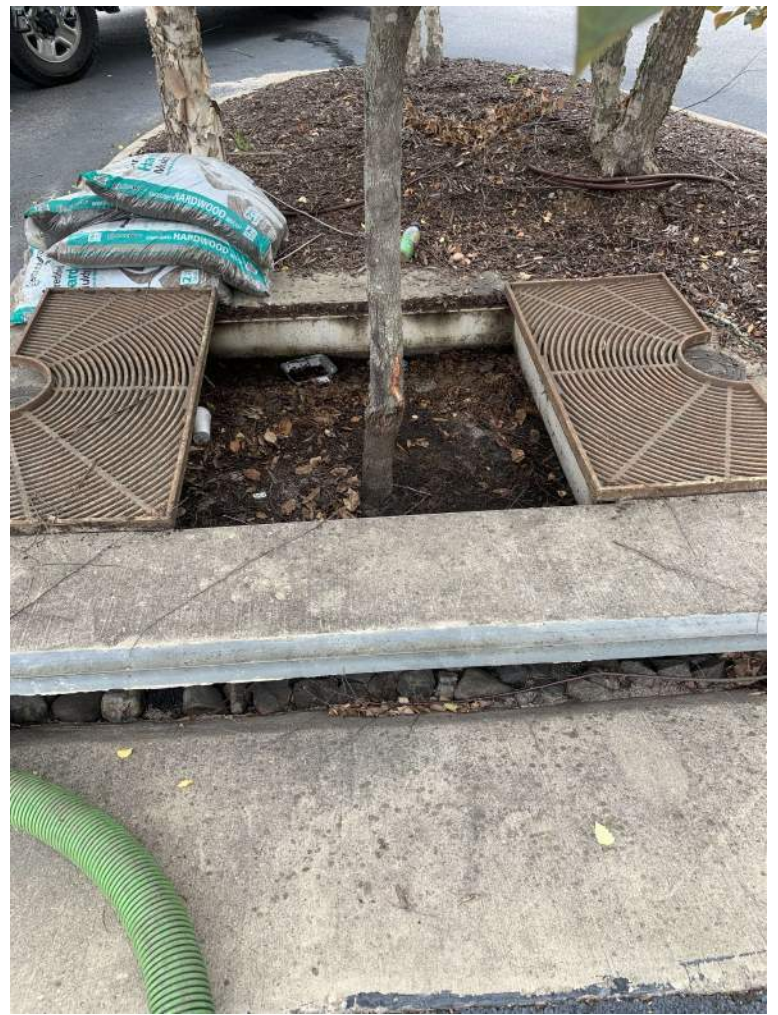
BMP #8- before maintenance
