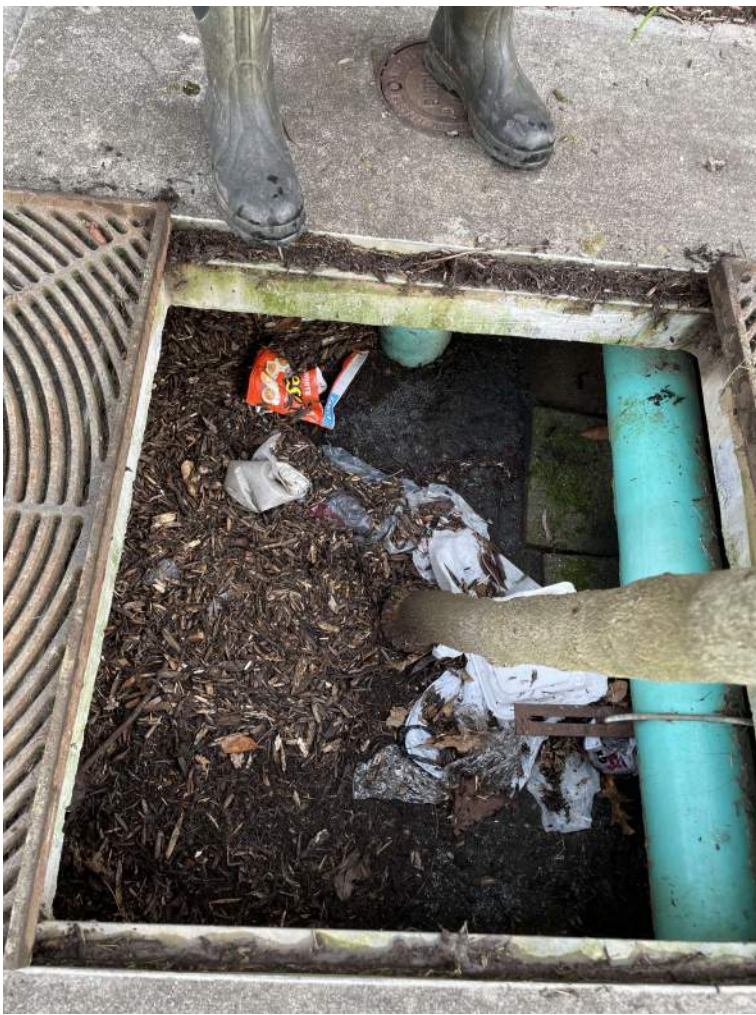
BMP #2- before maintenance
