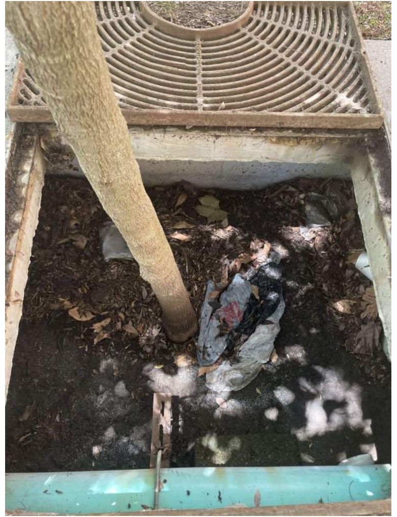
BMP#1- before maintenance
