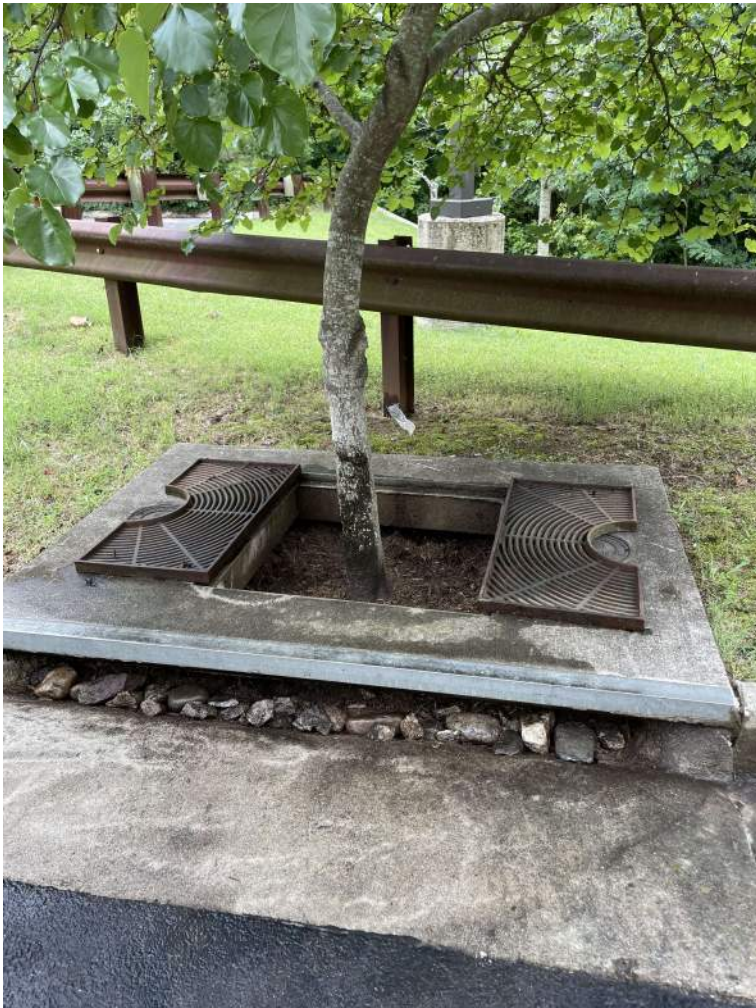
BMP #13- after maintenance
