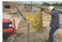
To clean Siltack® attach rebar through empty loops at bottom and lift to empty.
