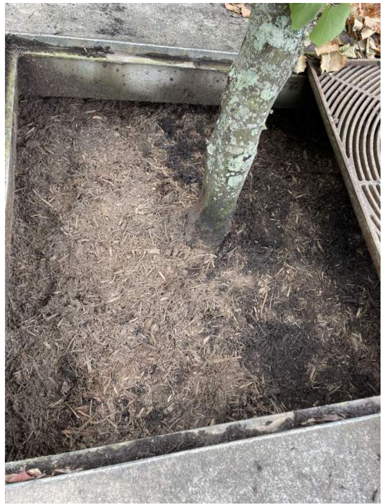
BMP #9- after maintenance
