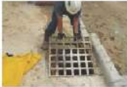
Remove grate from catch basin.
