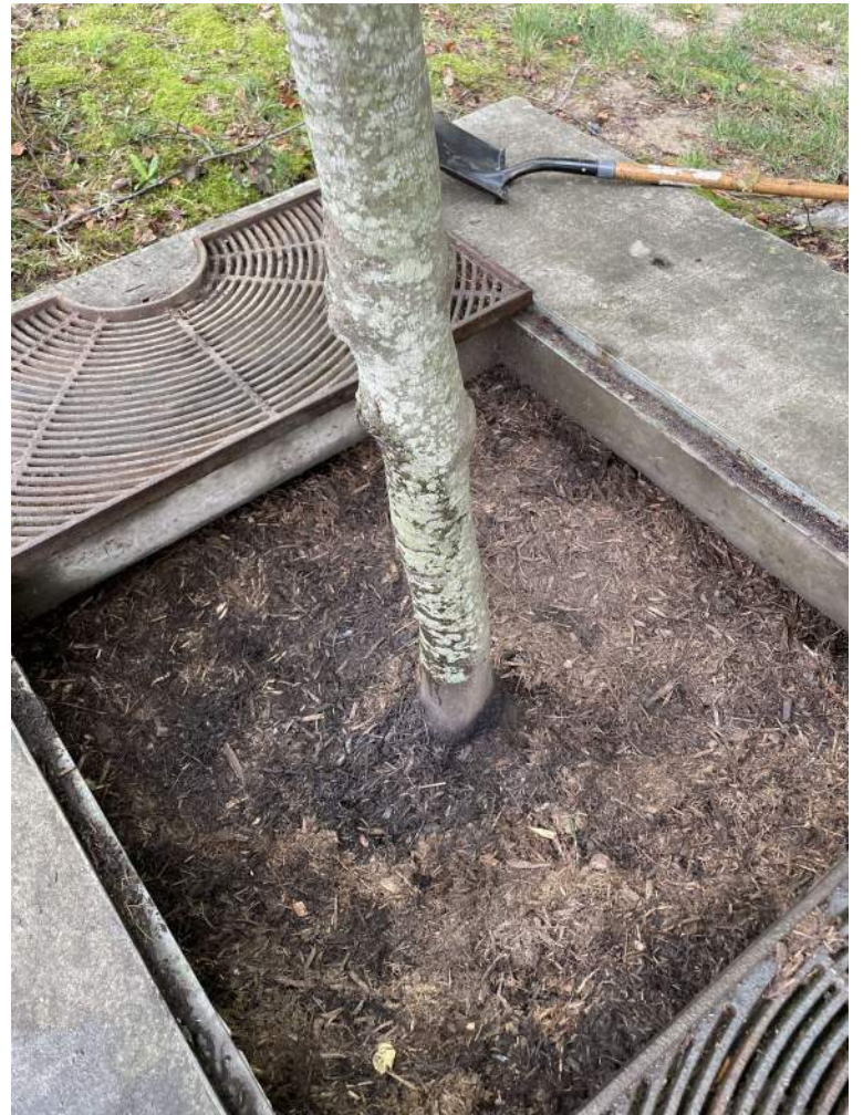
BMP #10- after maintenance
