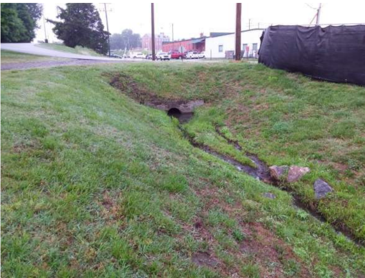
BMP #30- inlet channel
