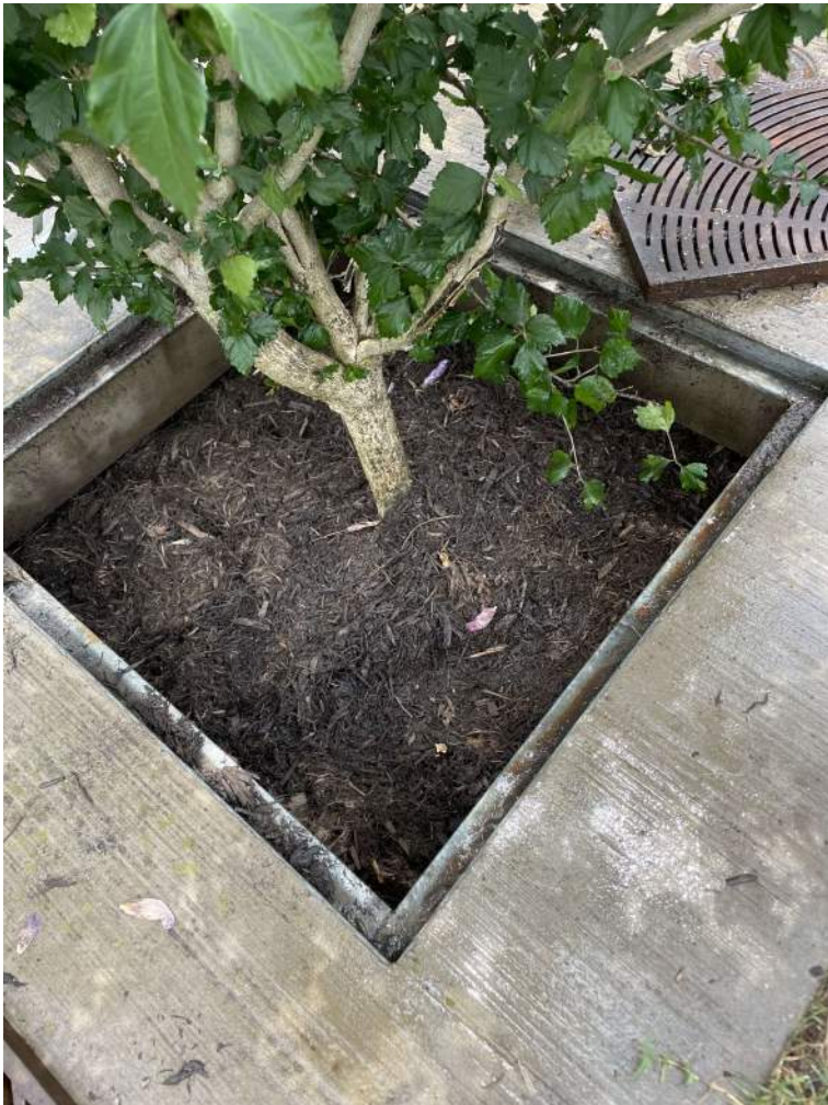
BMP #44- after maintenance
