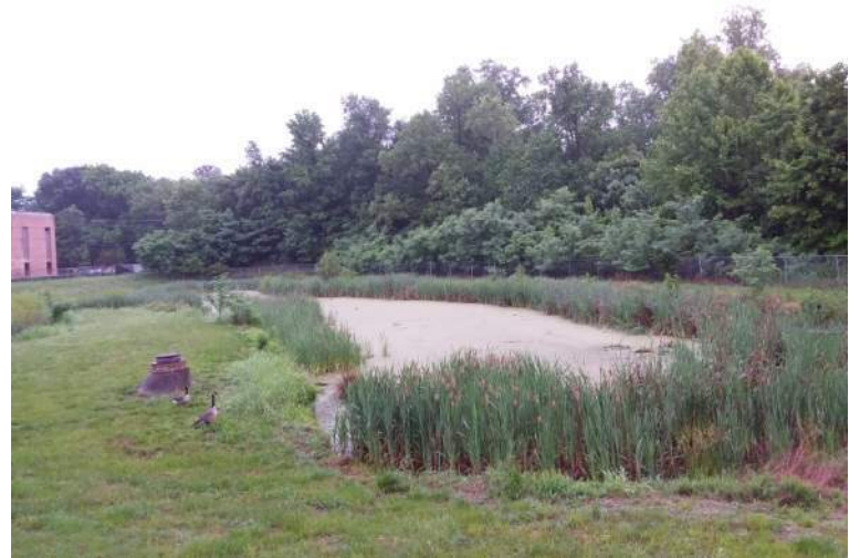
BMP #30- facing northwest
