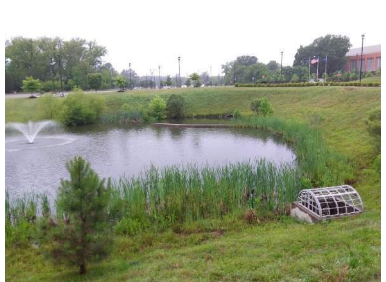
BMP #46- viewpoint looking towards outlet structure
