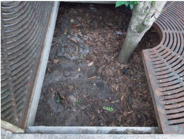
BMP #41- right side of filterra
