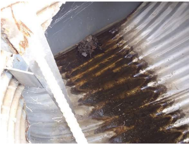
BMP #40- inside view of right manhole
