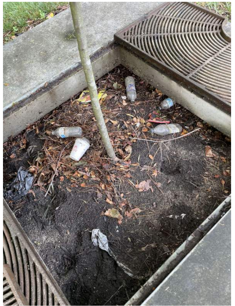
BMP #10- before maintenance
