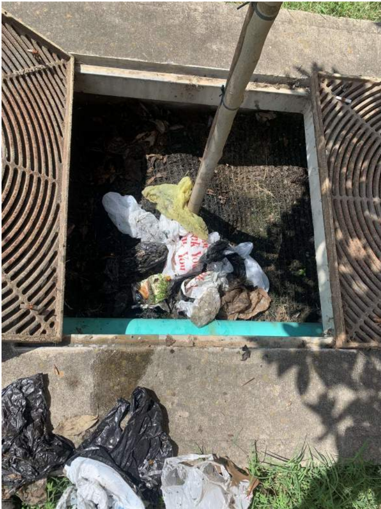
BMP #19- before maintenance
