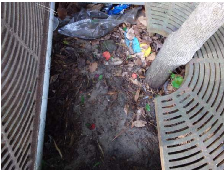
BMP #11- right side of filterra
