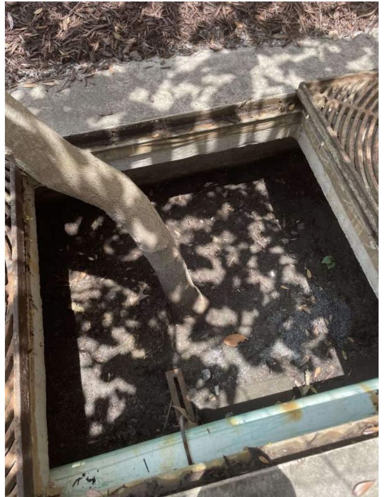
BMP #17- before maintenance
