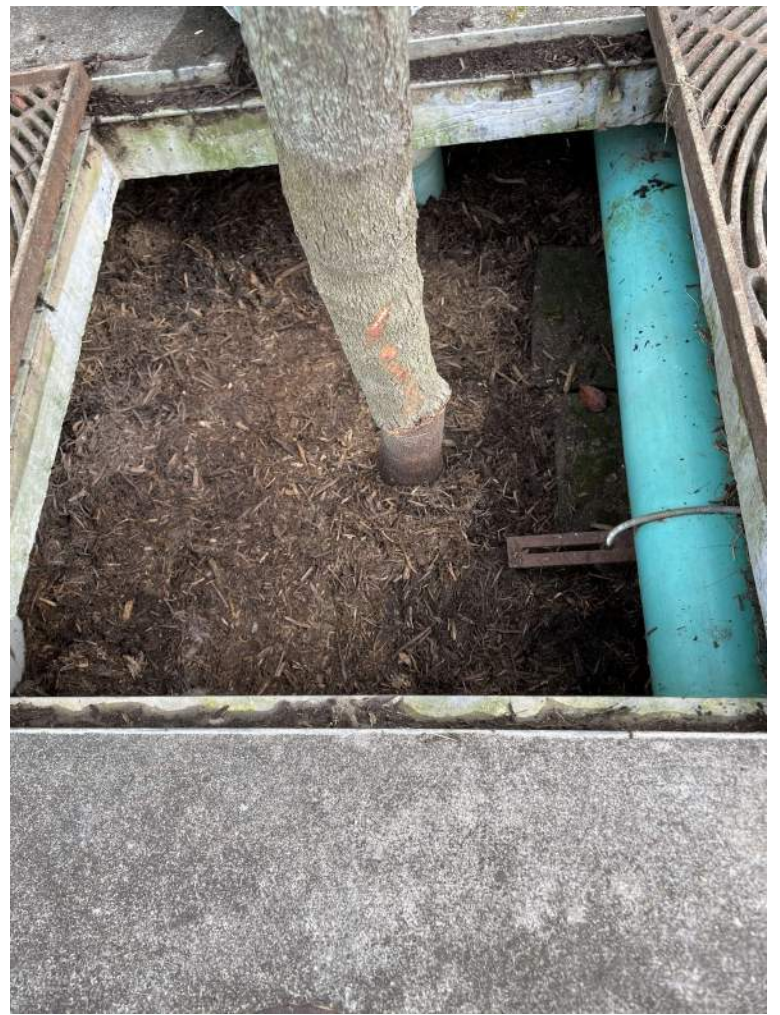
BMP #2- after maintenance
