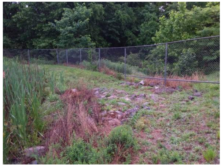
BMP #30- emergency spillway
