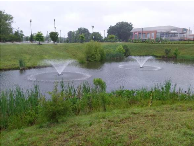
BMP #46- both fountains are operating properly
