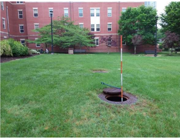
BMP #28- top view of detention chamber
