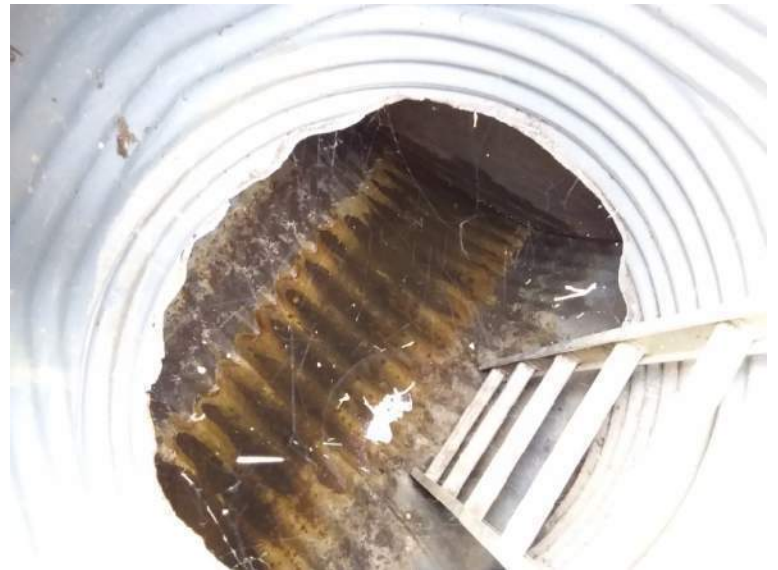
BMP #25- inside view of bottom manhole
