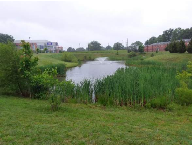
BMP #46- facing northwest
