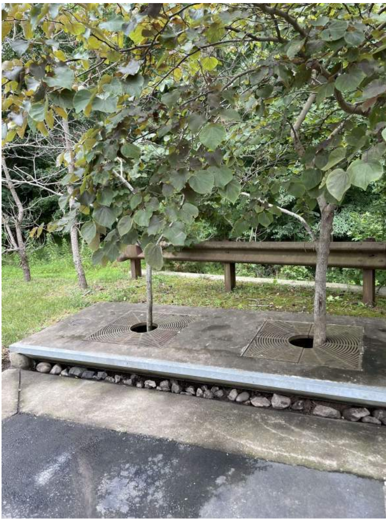
BMP #10- after maintenance
