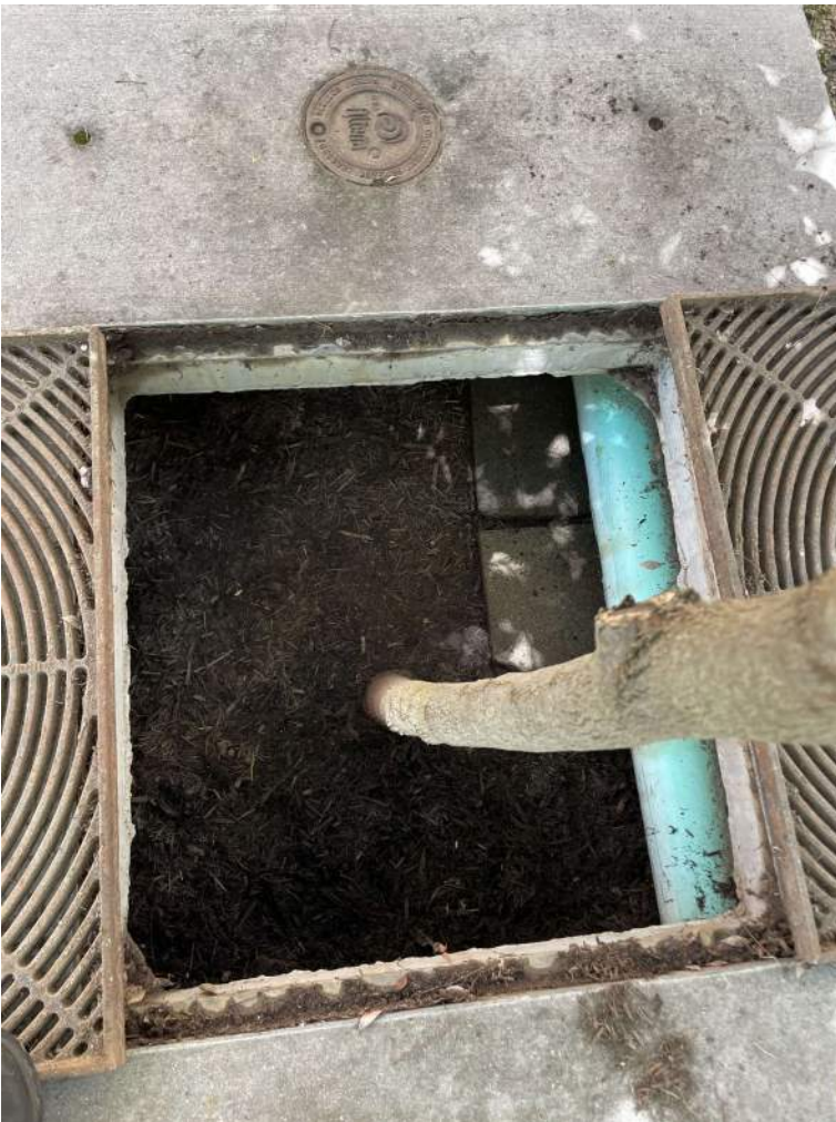
BMP #1- after maintenance
