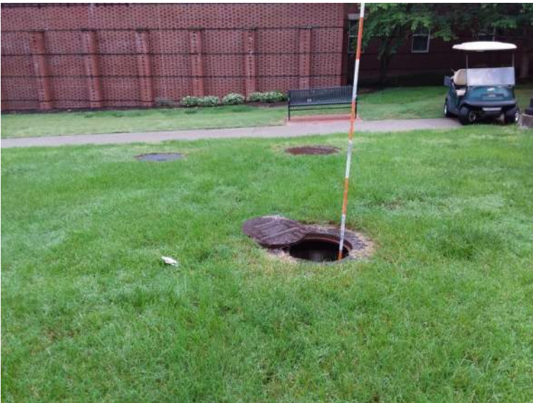
BMP #28- top view of sand filter side
