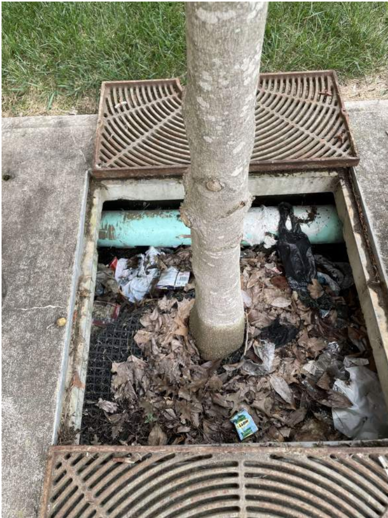
BMP #18- before maintenance
