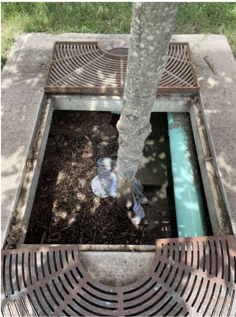
BMP #6- before maintenance
