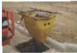
Removed Siltack® is now ready for cleanout.
