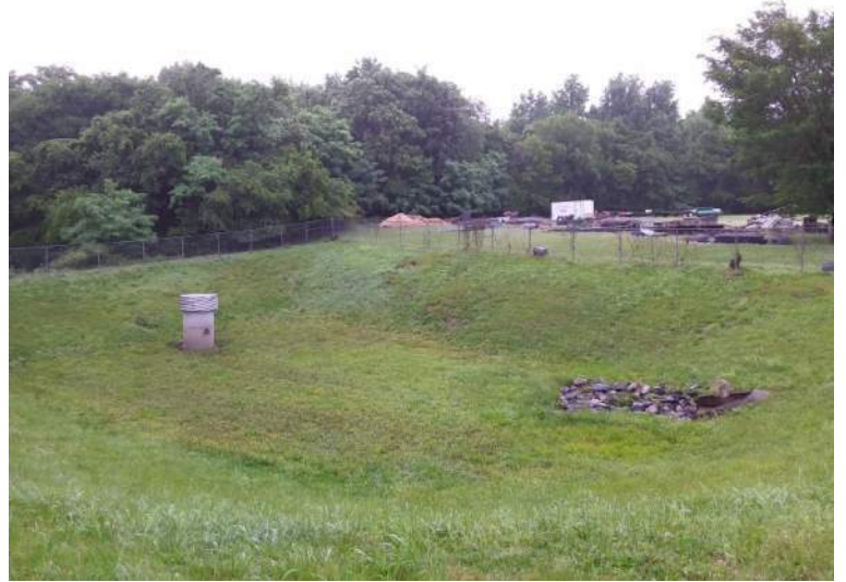
BMP #29- facing southwest
