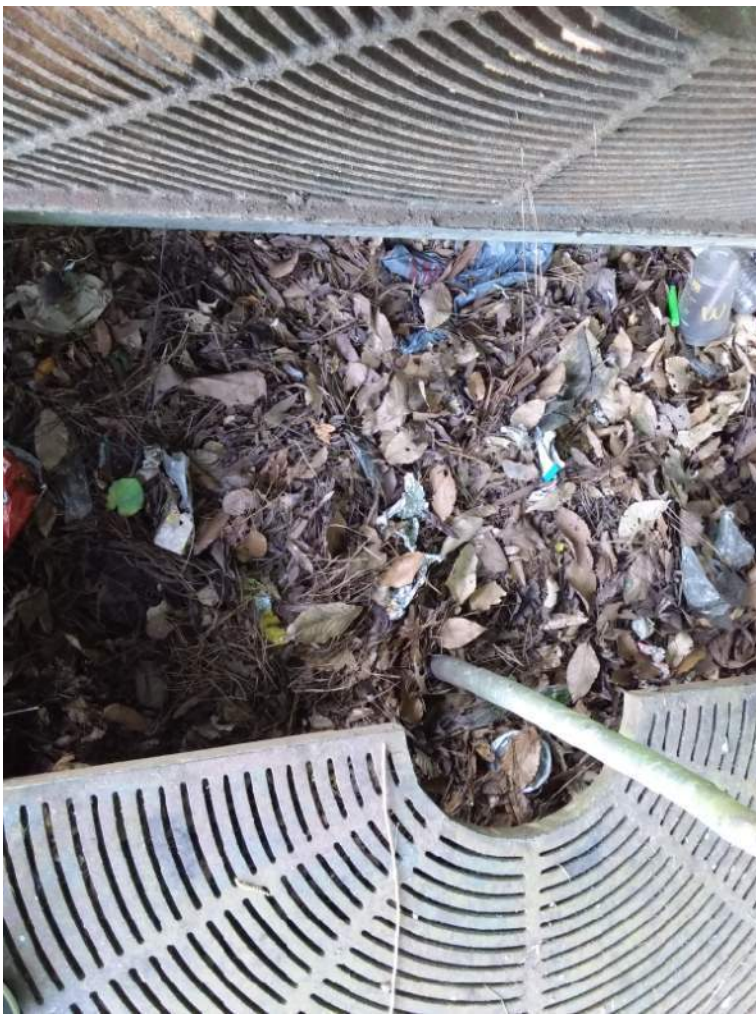
BMP #10- right side of filterra
