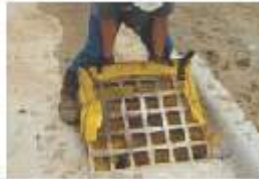
Slide Siltack® over one side of grate.
