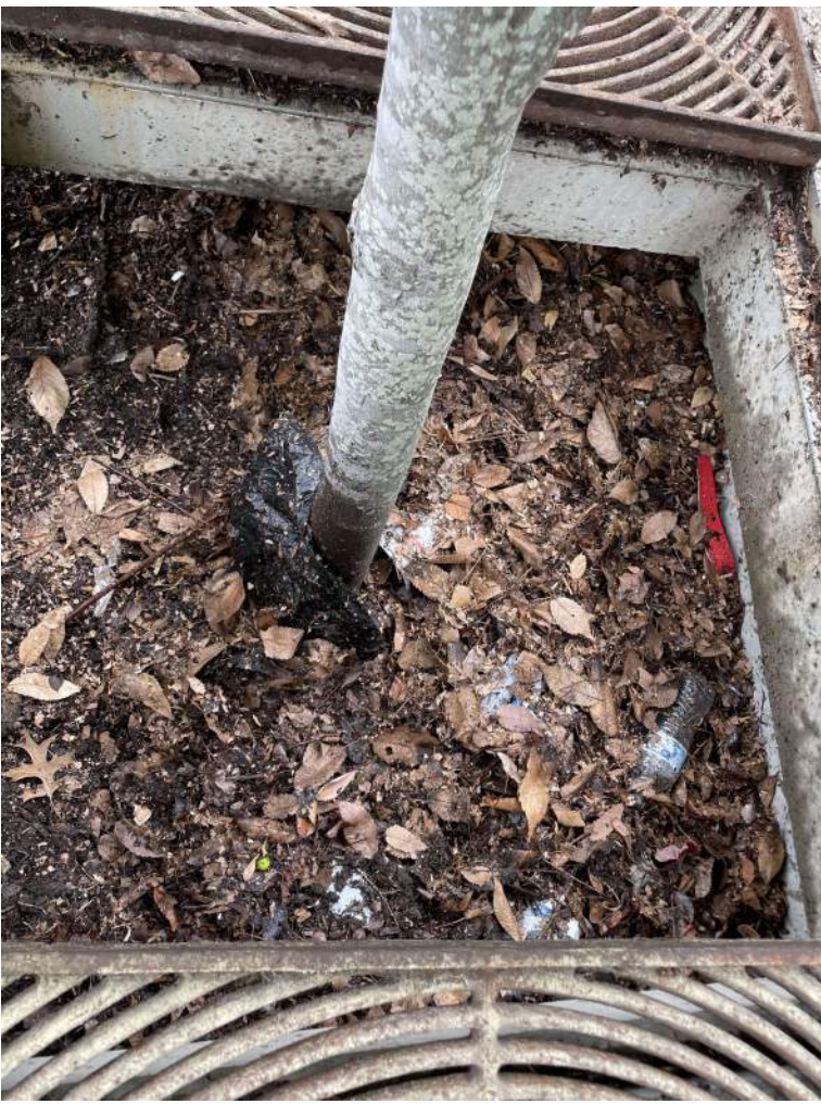
BMP #12- before maintenance
