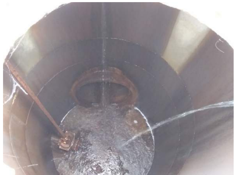
BMP #30- inside view of outlet structure
