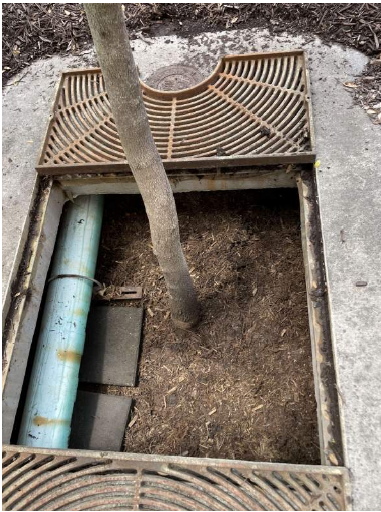
BMP #17- after maintenance
