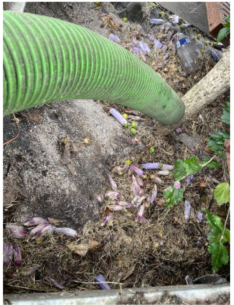
BMP #44- before maintenance
