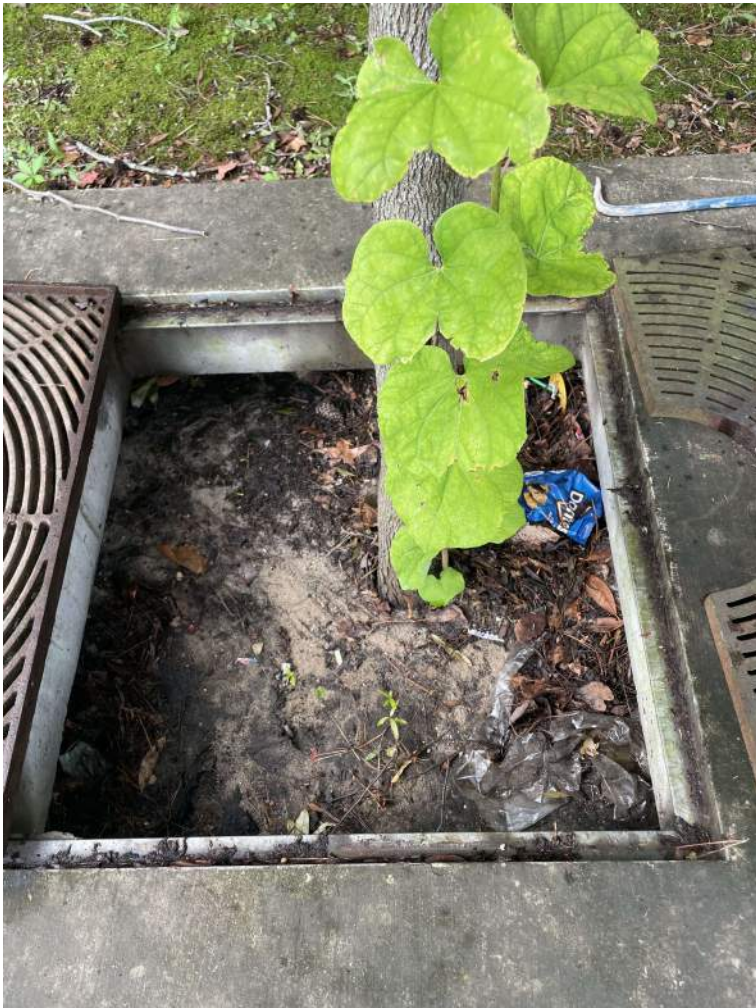
BMP #11- before maintenance
