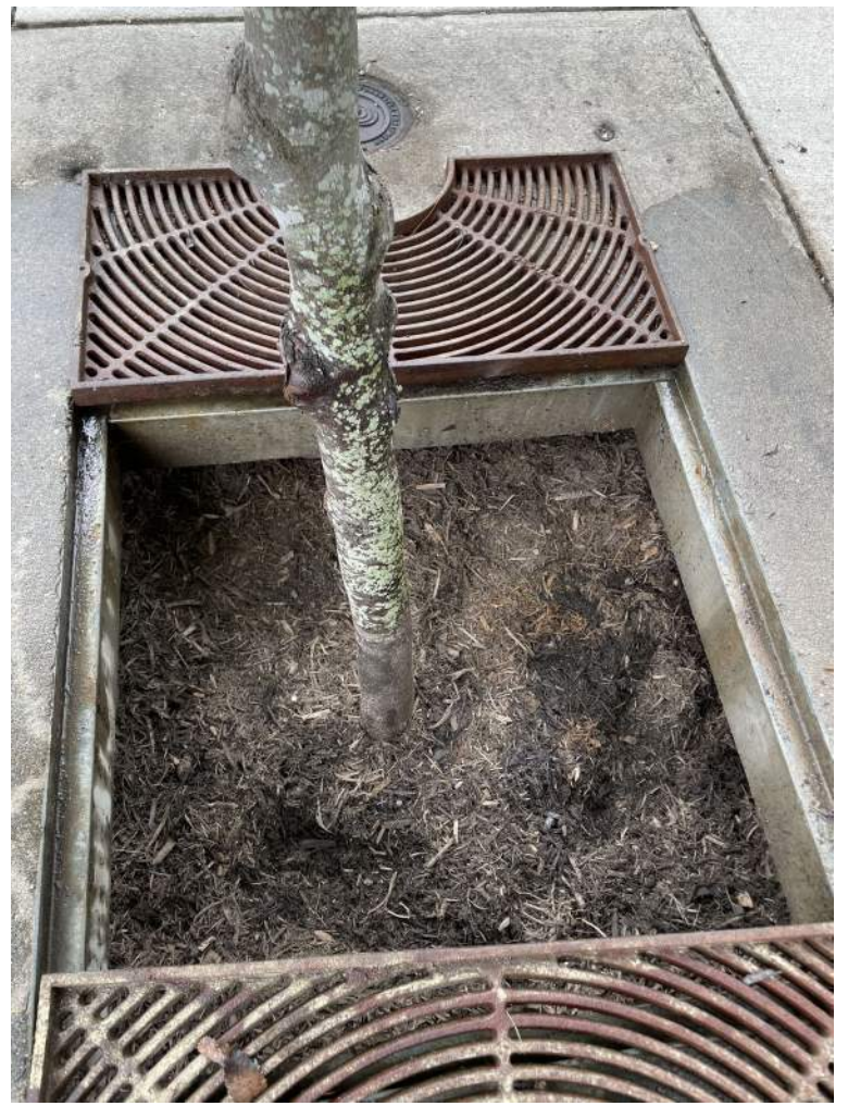
BMP #12- after maintenance
