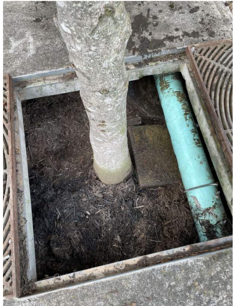
BMP #18- after maintenance
