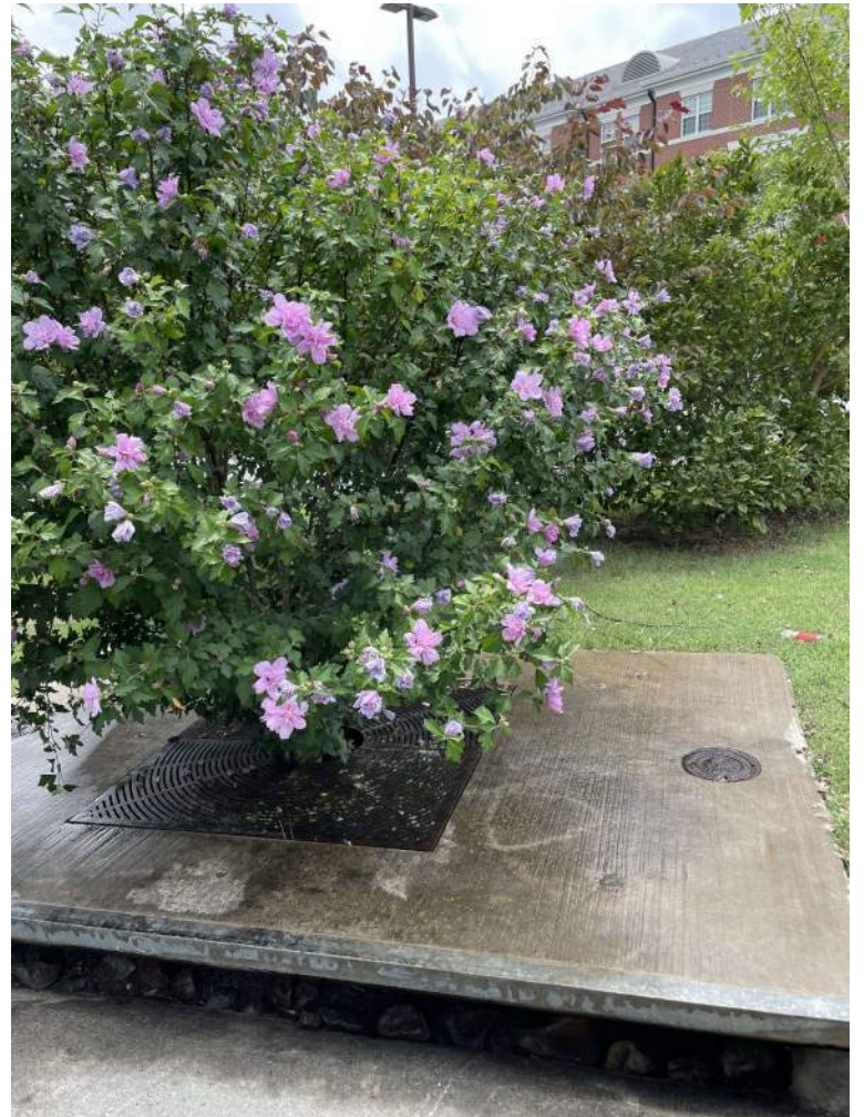
BMP #42- after maintenance
