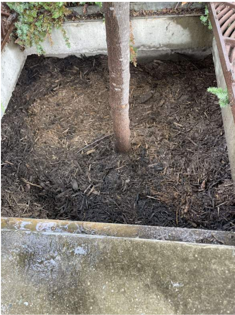
BMP #7- after maintenance
