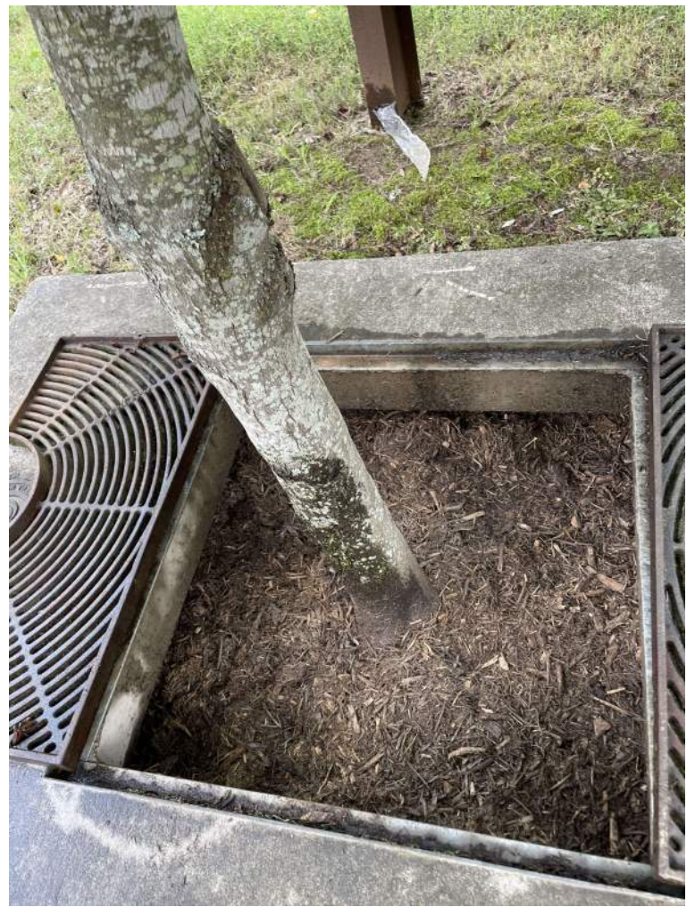
BMP #13- after maintenance
