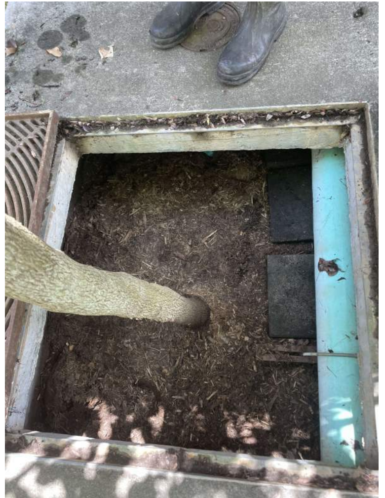
BMP #21- after maintenance
