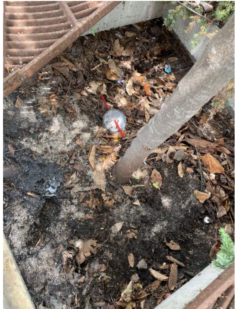
BMP #7- before maintenance
