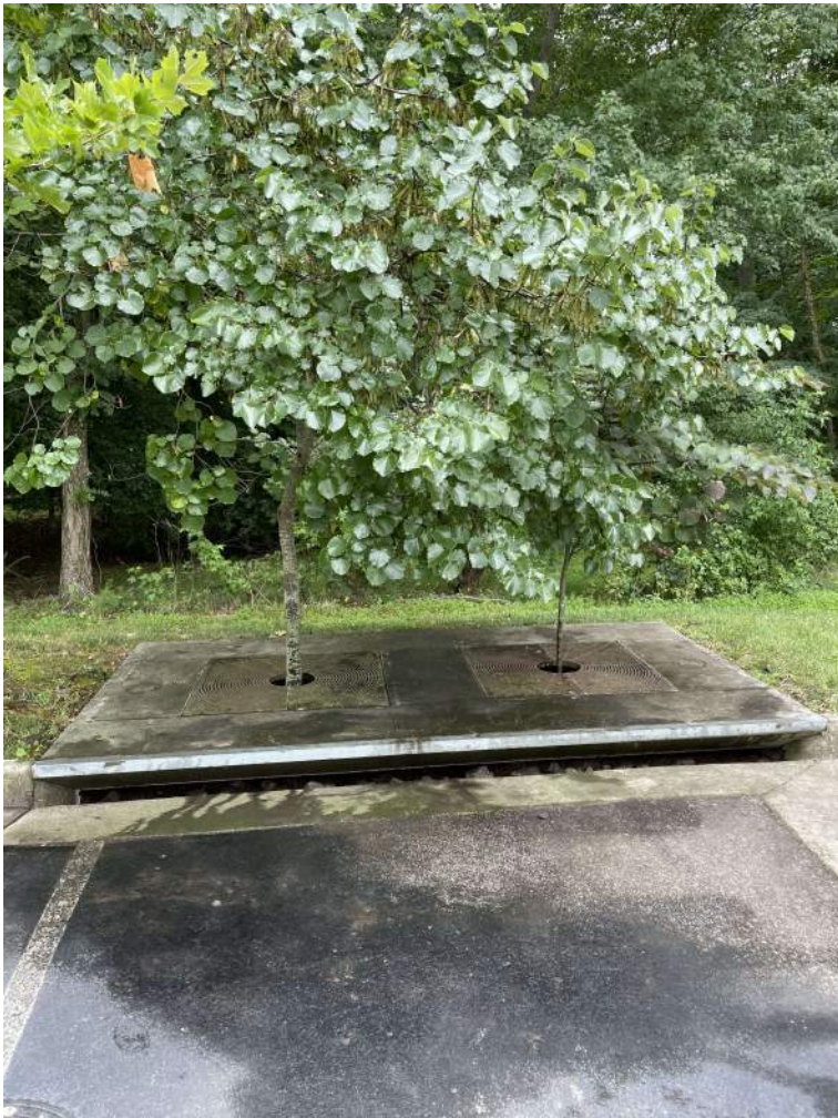
BMP #11- after maintenance
