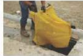
Slide Siltack® over opposite side of grate.
