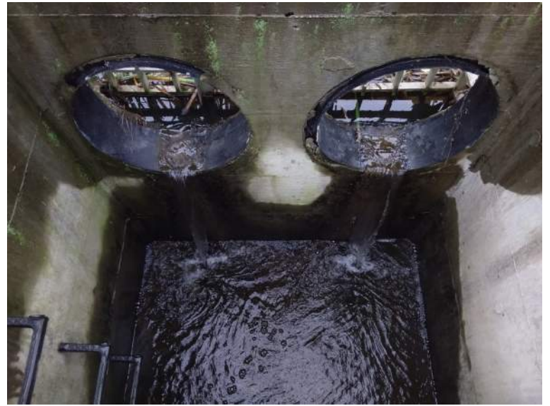
BMP #46- inside view of outlet structure
