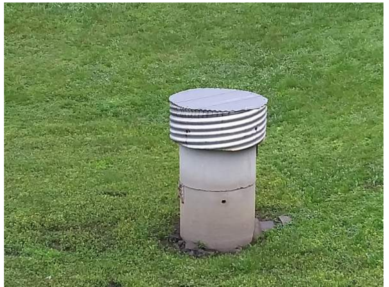
BMP #29- riser structure
