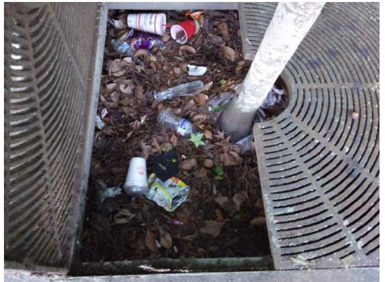
BMP #10- inside left side filterra
