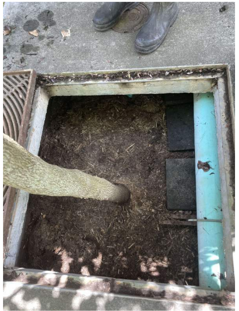
BMP #16- after maintenance
