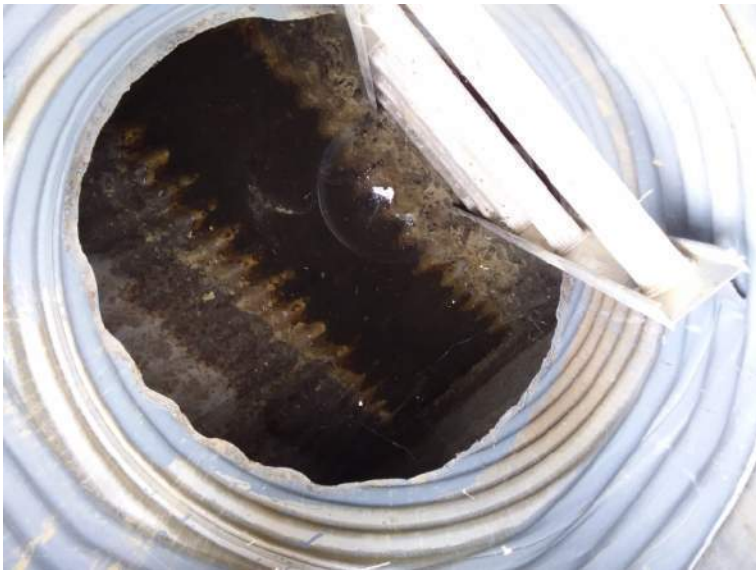
BMP #25- inside view of top manhole
