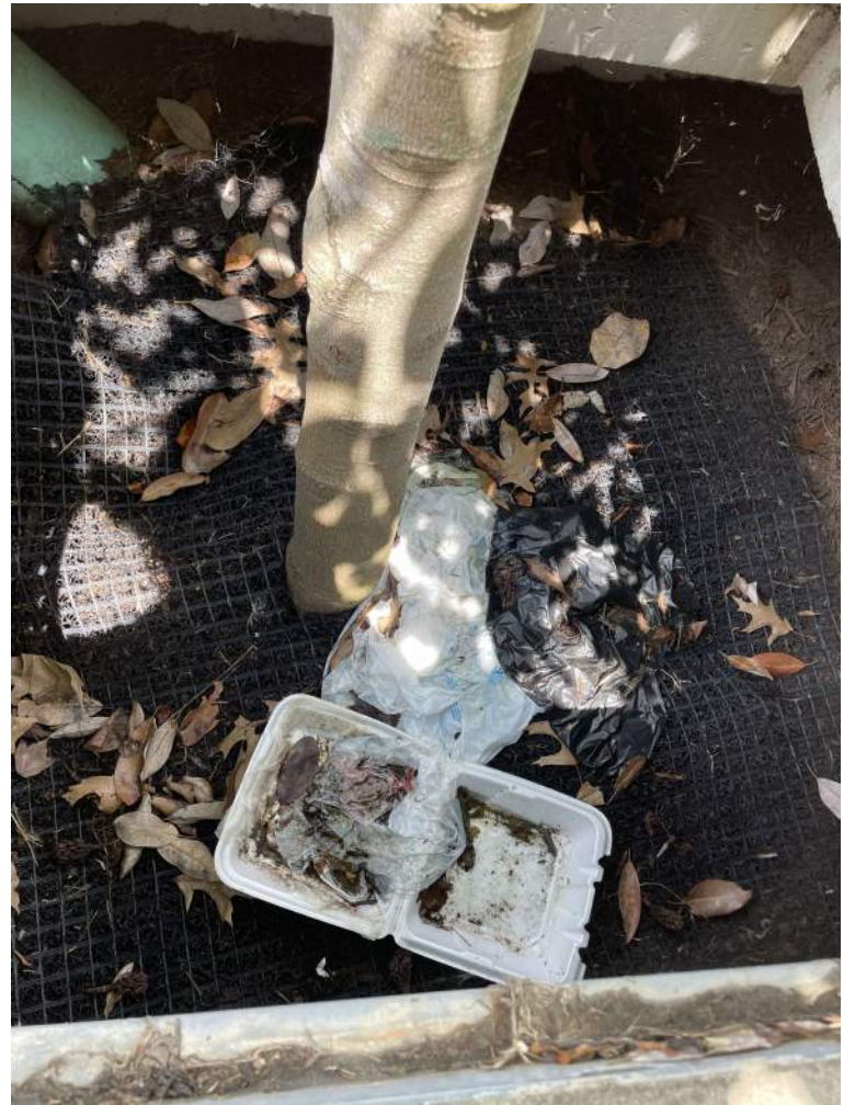
BMP #3- before maintenance
