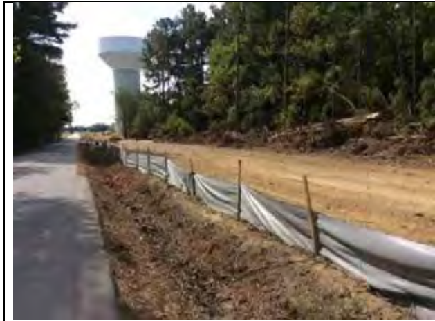
Stabilization needed
