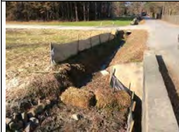
Remove silt fence from stream channel
