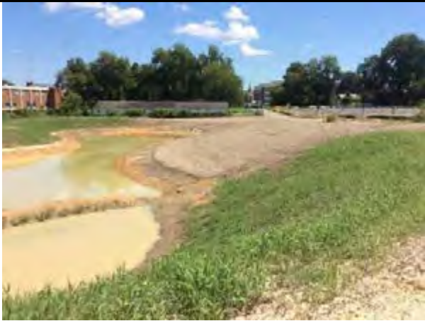
Stabilization needed
