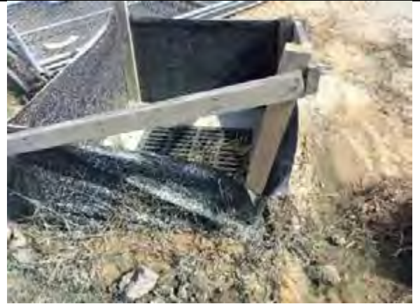
Repair inlet protection
