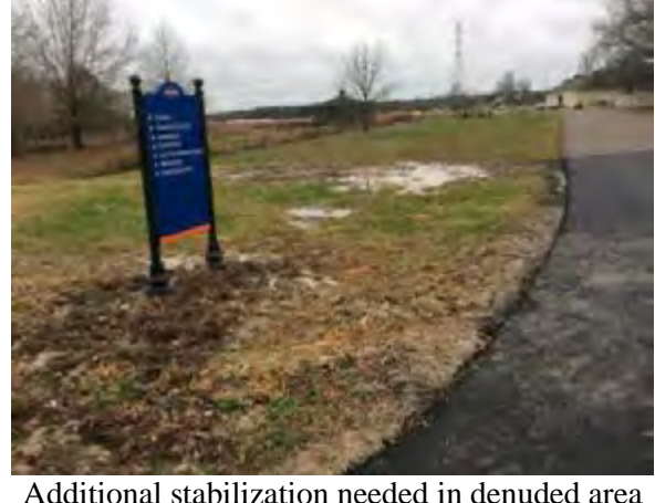
Additional stabilization needed in denuded area
