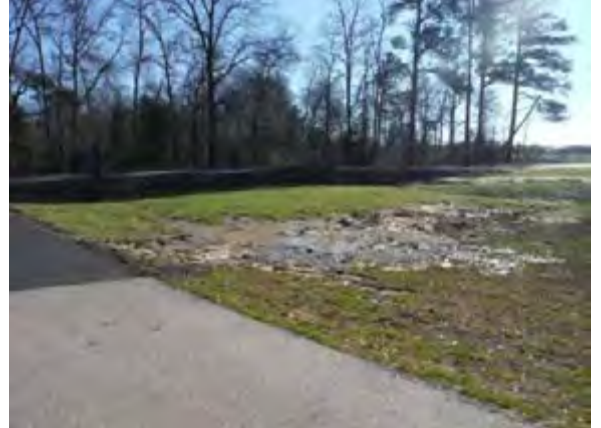
Additional stabilization needed in denuded area
