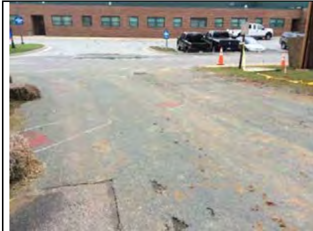
Sediment tracking in roadway
