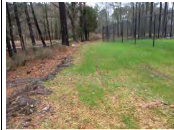
Additional stabilization needed in denuded area
