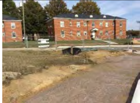
Repair inlet protection
