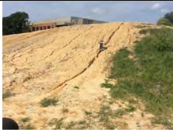
Stabilization needed and rill repair
