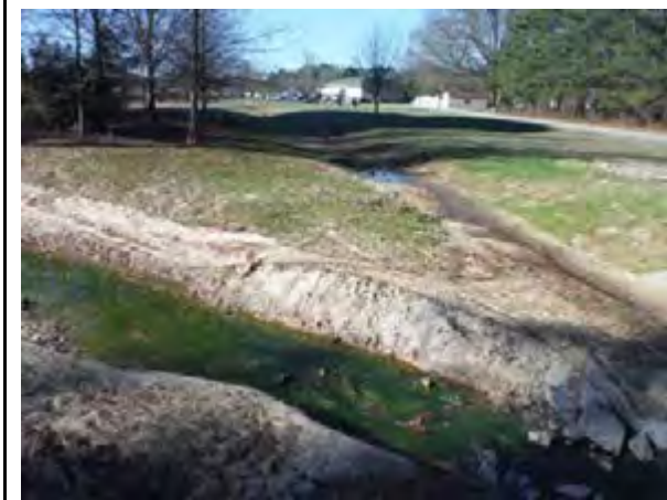
Additional stabilization needed in denuded area
