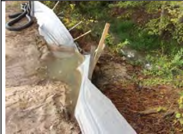
Repair silt fence
