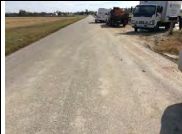
Sediment tracking in road
