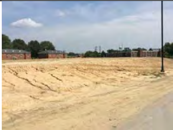
Stabilization needed and rill repair
