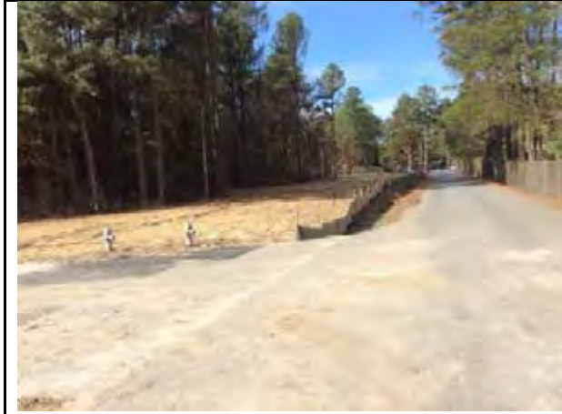
Sediment tracking in road
