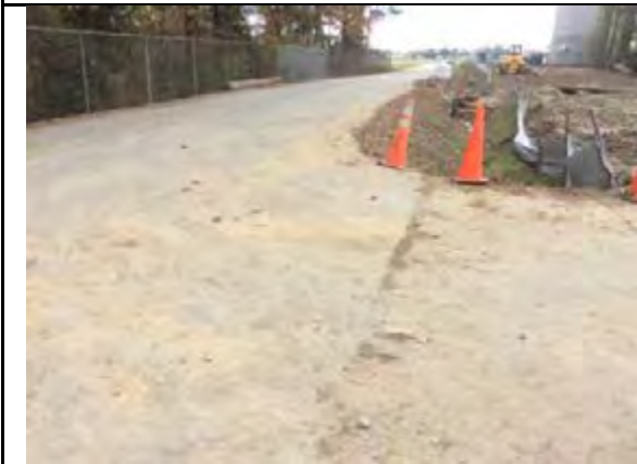
Sediment tracking in road
