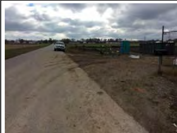
Sediment tracking in road
