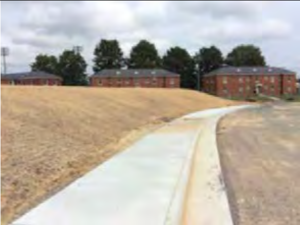
Stabilization needed and rill repair
