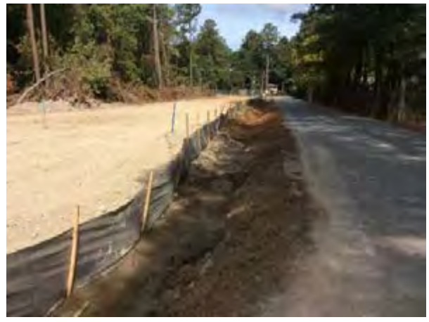
Stabilization needed
