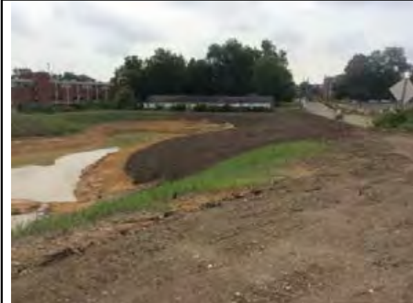
Stabilization needed
