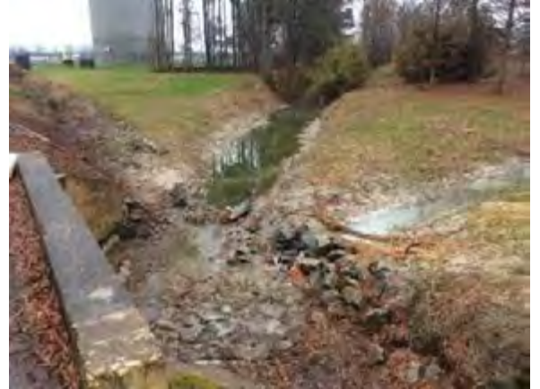
Additional stabilization needed
