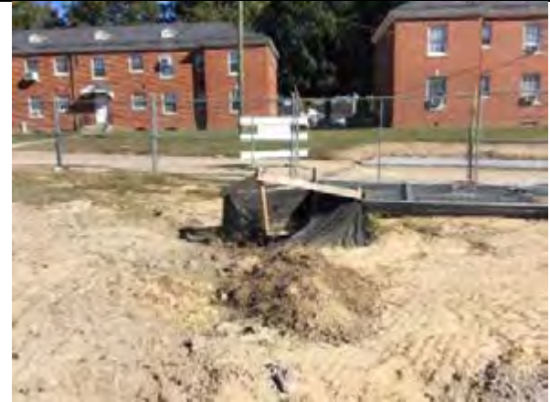
Repair inlet protection
