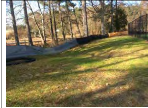
Remove silt fence
