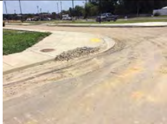
Clean out inlet protection
