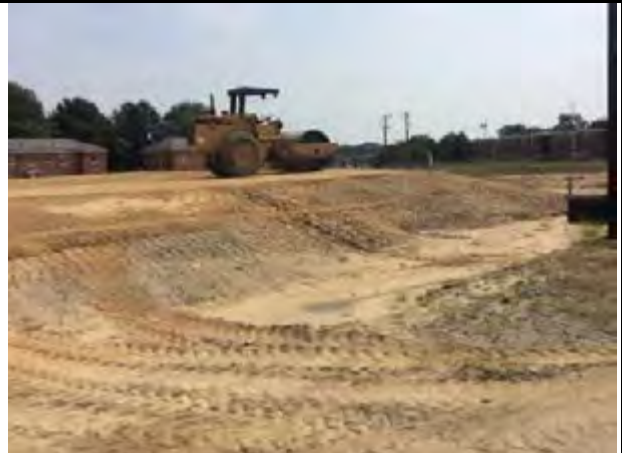
Stabilization needed and rill repair
