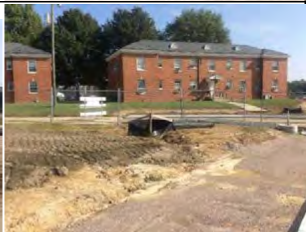
Repair inlet protection
