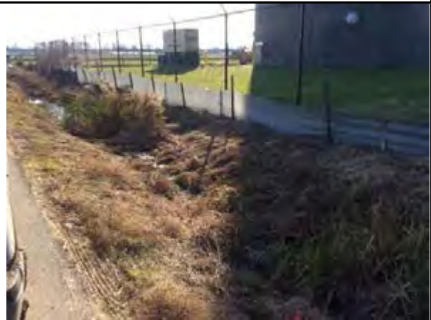
Remove silt fence
