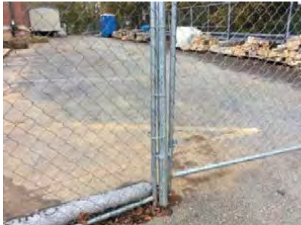
Sediment tracking in roadway
