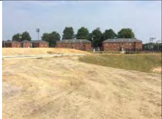
Stabilization needed
