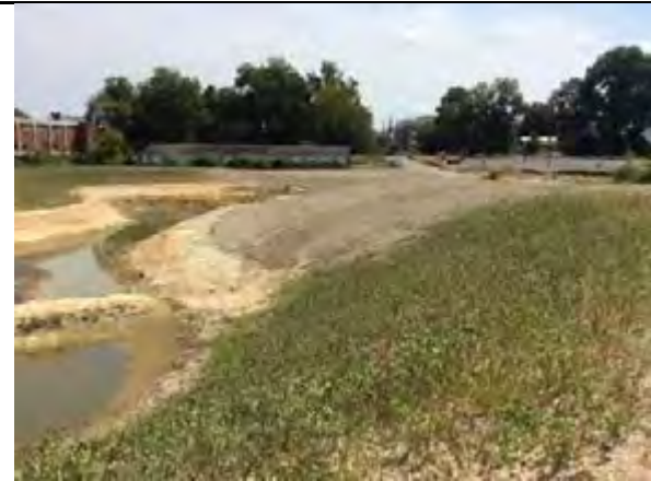
Stabilization needed
