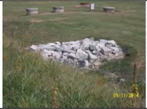
Fig. 2 – Check dam along east side of building that requires shaping revisions (view-east).
