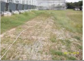
Fig. 4 – Continue to water areas where new EC mat has been installed around the building (view-east).
