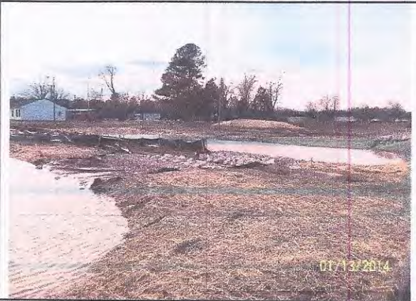
Fig. 6 – Temporary sediment trap #4 and outlet protection (view-northwest).
