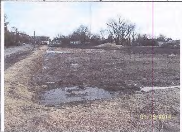
Fig. 4 – Apply temporary seeding to all denuded areas (view-south).
