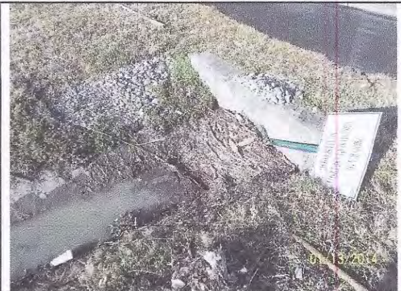
Fig. 2 – Remove debris from all storm pipe inlets to promote drainage (view-northeast).
