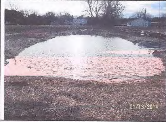
Fig. 5 – Temporary sediment trap #5 (view-west).
