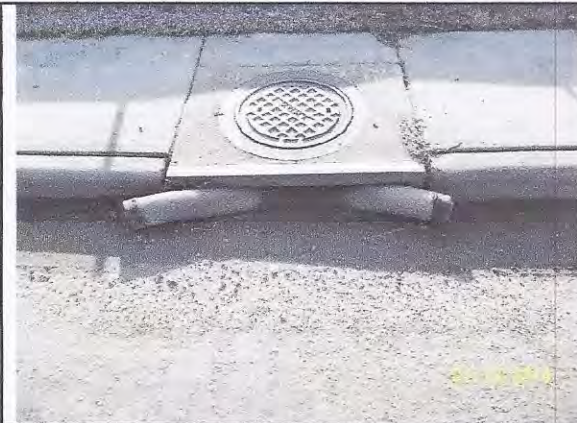
Fig. 1 – Remove sediment from roadway inlets and reinstall inlet protection (view-west).
