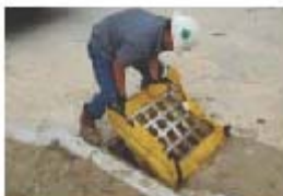
Replace Siltsock® and grate inlet into recess.
