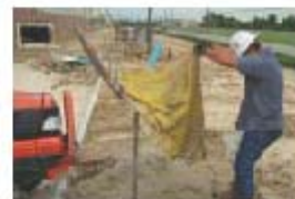
To clean Siltsock® attach rebar through empty loops at bottom and lift to empty.
