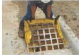
Slide Siltsock® over one side of grate.
