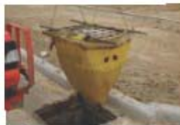
Removed Siltsock® is now ready for cleanout.
