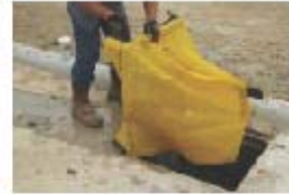
Slide Siltsock® over opposite side of grate.
