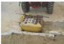
Slowly remove Siltsock® from inlet.
