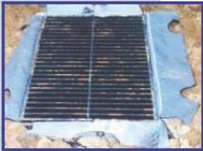
installed Siltsack held in place by grate.
