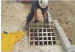
Remove grate from catch basin.
