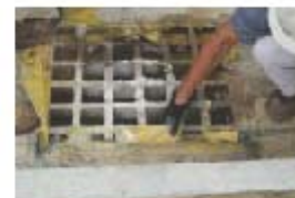
To remove Siltsock®, clean area around grate and slide rebar through Siltsock® pockets.
